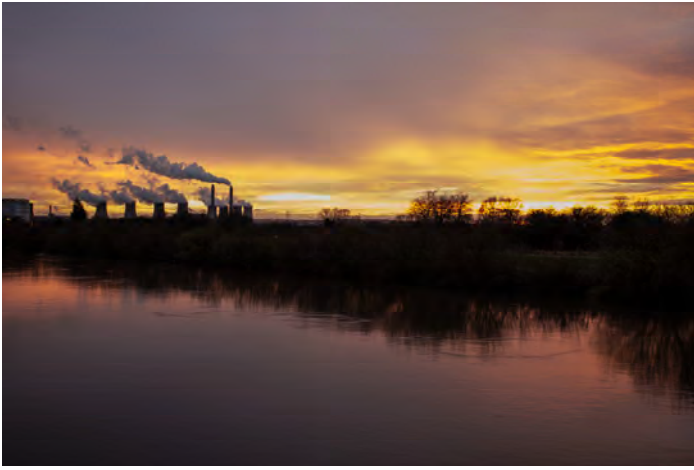
The cooling towers at the West Burton Power Station. Image courtesy of Stephen Teather.
