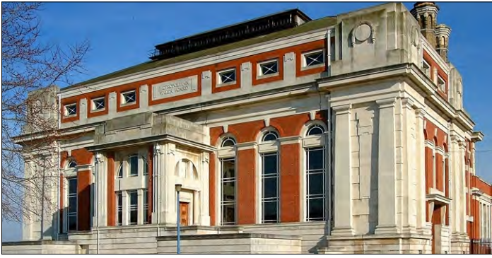
Kempton II pumping station. Image copyright James Douet.
