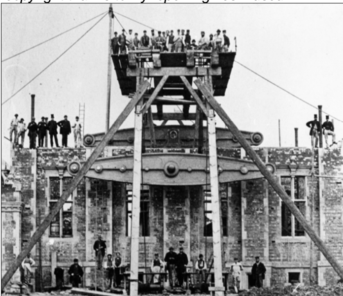
Ryhope Pumping Station during construction. Image copyright thanks to Ryhope Engines Museum.
