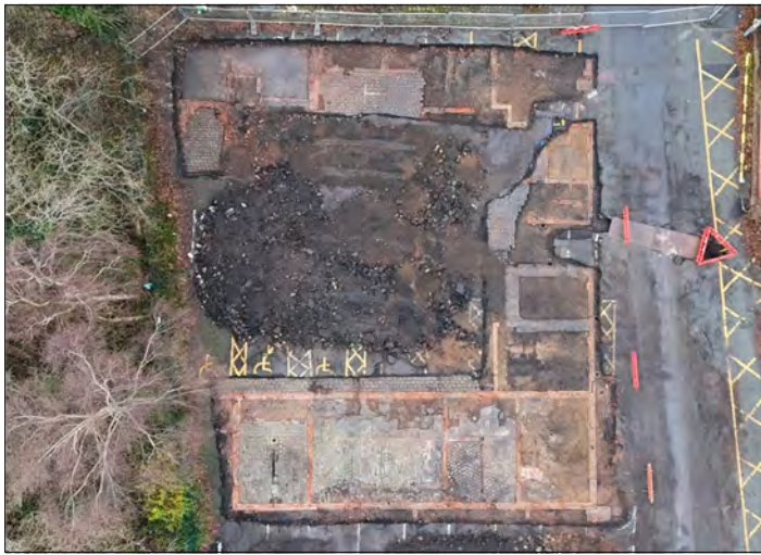
Drone Photograph of the excavated remains at Prestwich Fire Station. Image courtesy of Civic Heritage.
