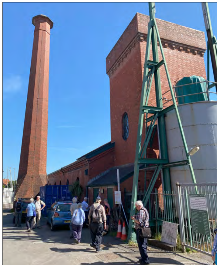
Hydraulic engine house, Underfall Yard. Copyright: Bill Barksfield.
