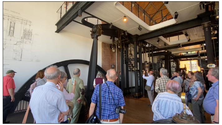
One of four engines on view at the Barbadinhos steam pumping station. Copyright Bill Barksfield.
