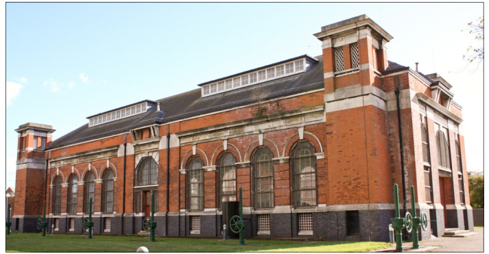
George V pumping station (1913). Courtesy of the Historic England Archive
