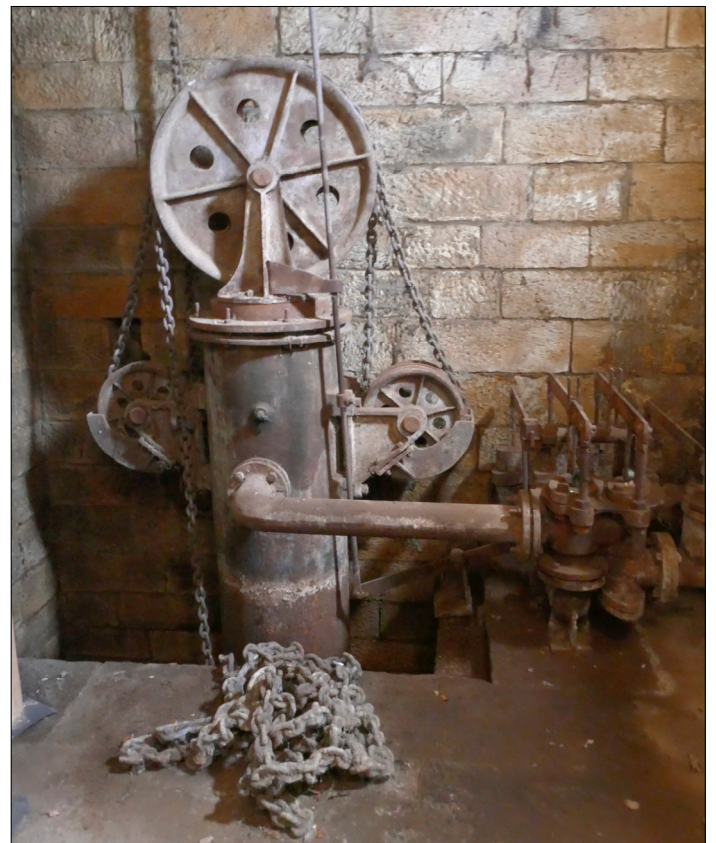
The Cragend hydraulic machinery in the silo. Copyright Lou Renwick.
