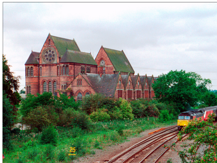
The two engine houses at Whitacre (1871-84). Courtesy of the Historic England Archive.
