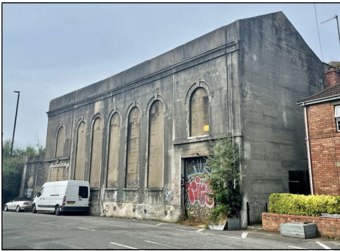
Avon Crescent substation, Underfall, Bristol. Image copyright Betty Woolerton
