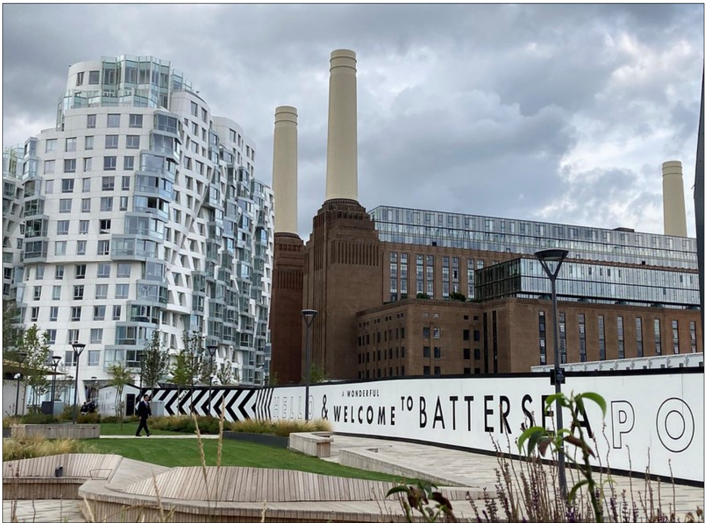
The restored Battersea Power Station. Image copyright Matt Brown.
