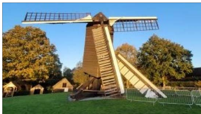
Nutley Windmill damage. Image copyright: Uckfield & District Preservation Society.
