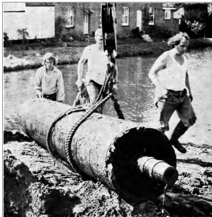
The Archimedes screw was rediscovered in 1973 during dredging and restoration of the Hungerford Basin (image courtesy of Crofton Beam Engines).
