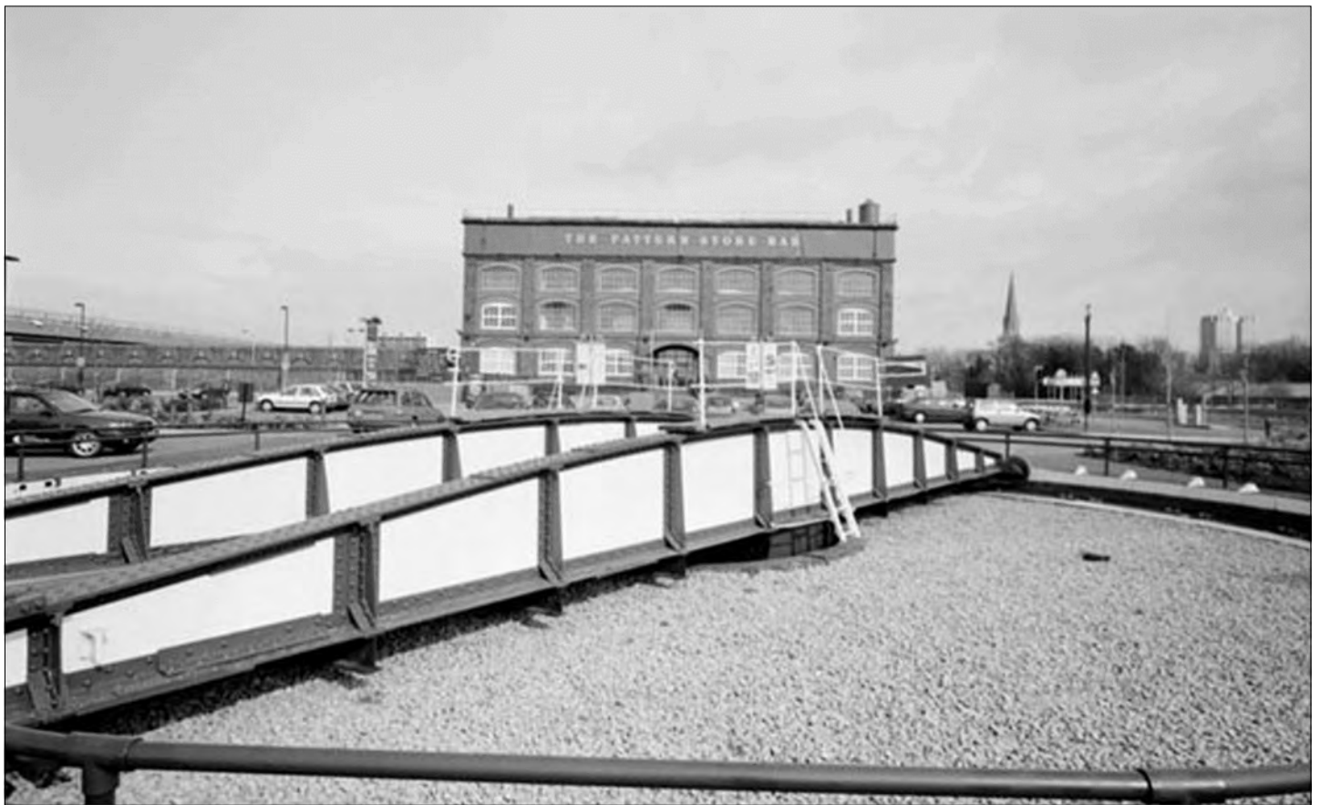
The Pattern Store, Swindon, with the listed railway turntable in the foreground. Image courtesy of Historic England.
