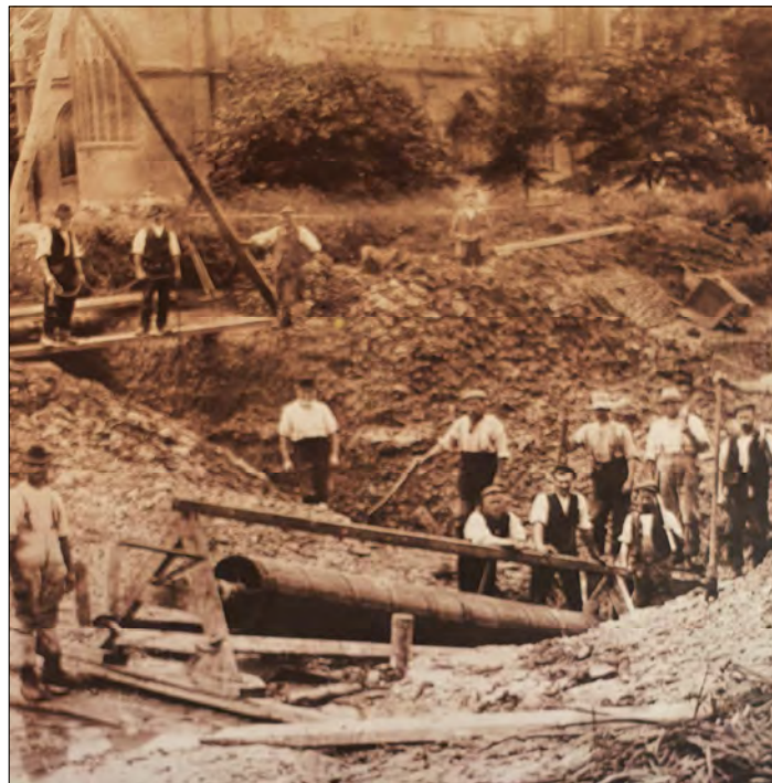
The Archimedes screw during maintenance at Hungerford Basin, Kennet & Avon Canal (image courtesy of Crofton Beam Engines).
