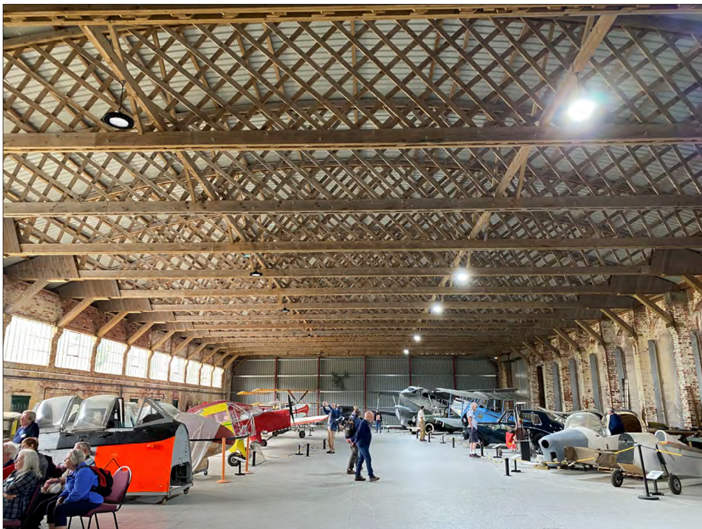
The 80ft span Belfast Truss at Hooton Park. Copyright Bill Barksfield.
