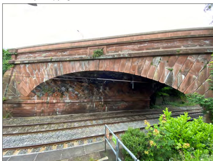
Sandstone 34° skew bridge at Rainhill No 762 Wirral Tramway. Copyright: Bill Barksfield.
