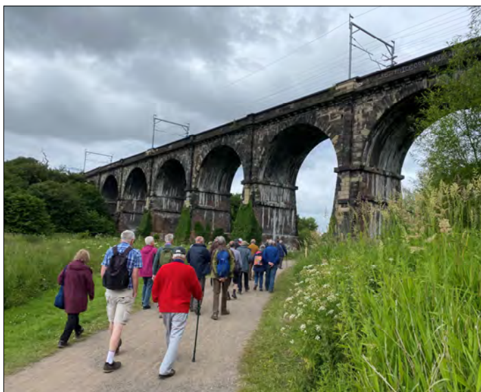
1830 Nine arch Sankey Viaduct with the AIA delegates below. Copyright: Bill Barksfield.
