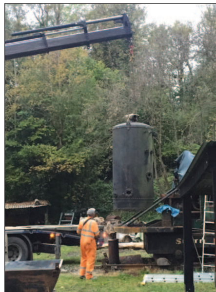
The boiler being lifted off – October 2021
