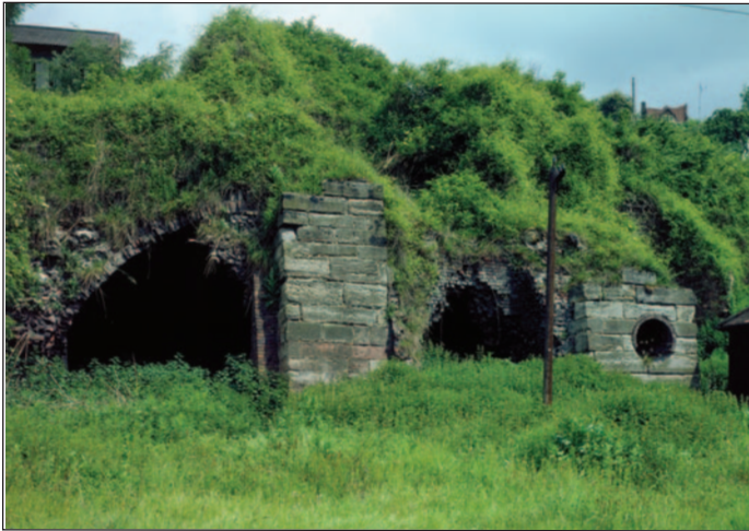
Bedlam furnace in 1969, before excavation.
