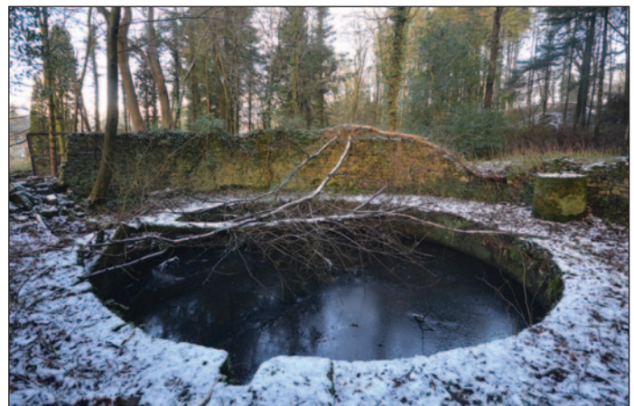
Remains of the gas holder tank at Dolphinhholme Worsted Mill © Matt Bristow, Historic England.
