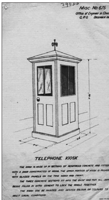
Fig 1. Drawing of concrete type Kiosk No 1
