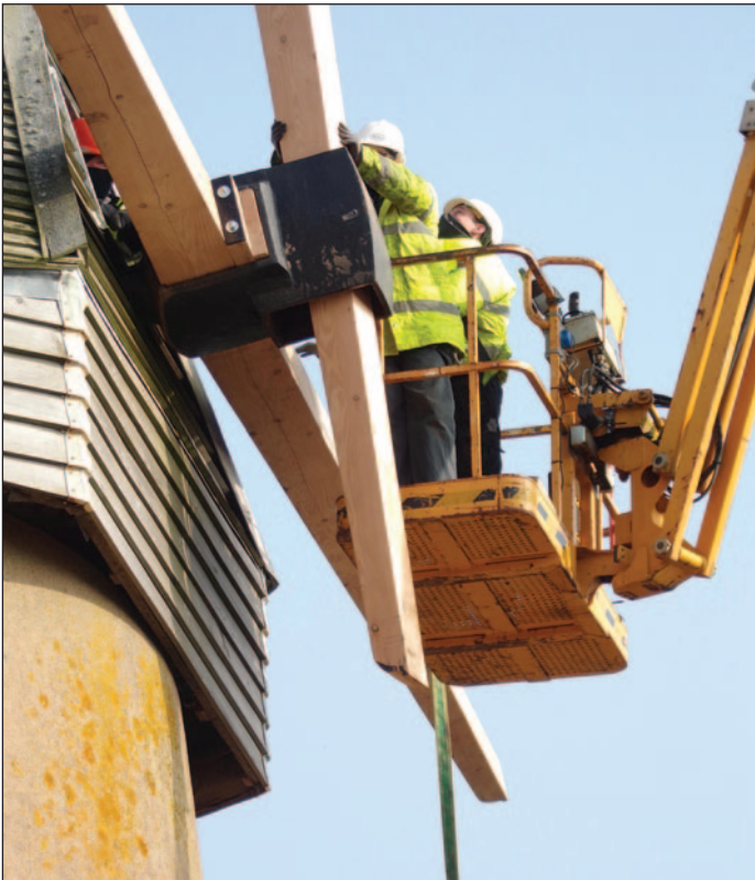
The stocks are wedged into the windshaft
