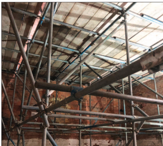
Bird cage scaffold in place
