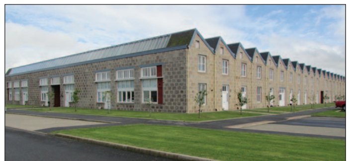
Inverurie Carriage Works
