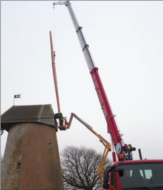
A rough-terrain crane hoisted the components
