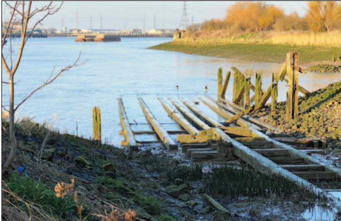
The slipway at Woolwich Arsenal after clearance of dense vegetation, February 2021
