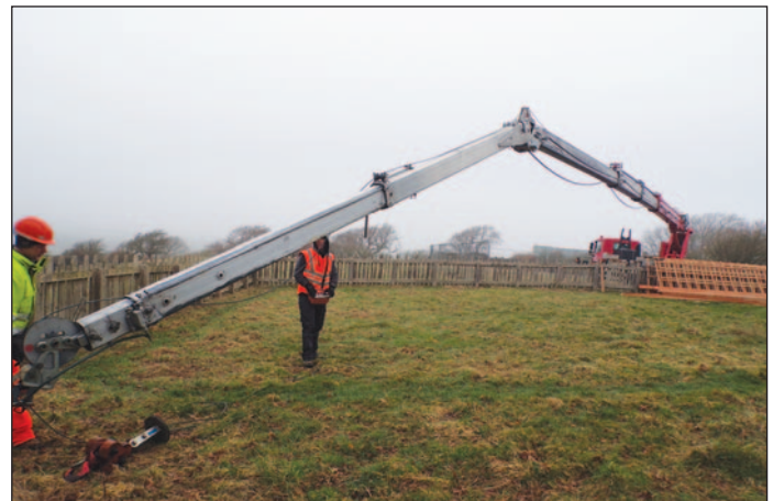
Rigging the crane
