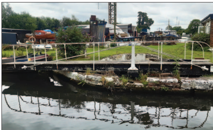
Swing bridge before restoration
