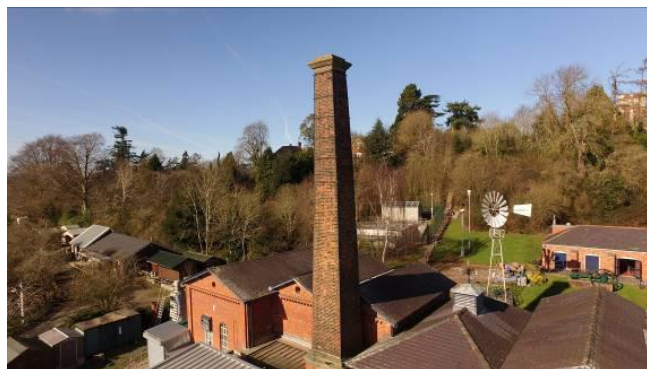
Hereford Waterworks Chimney
