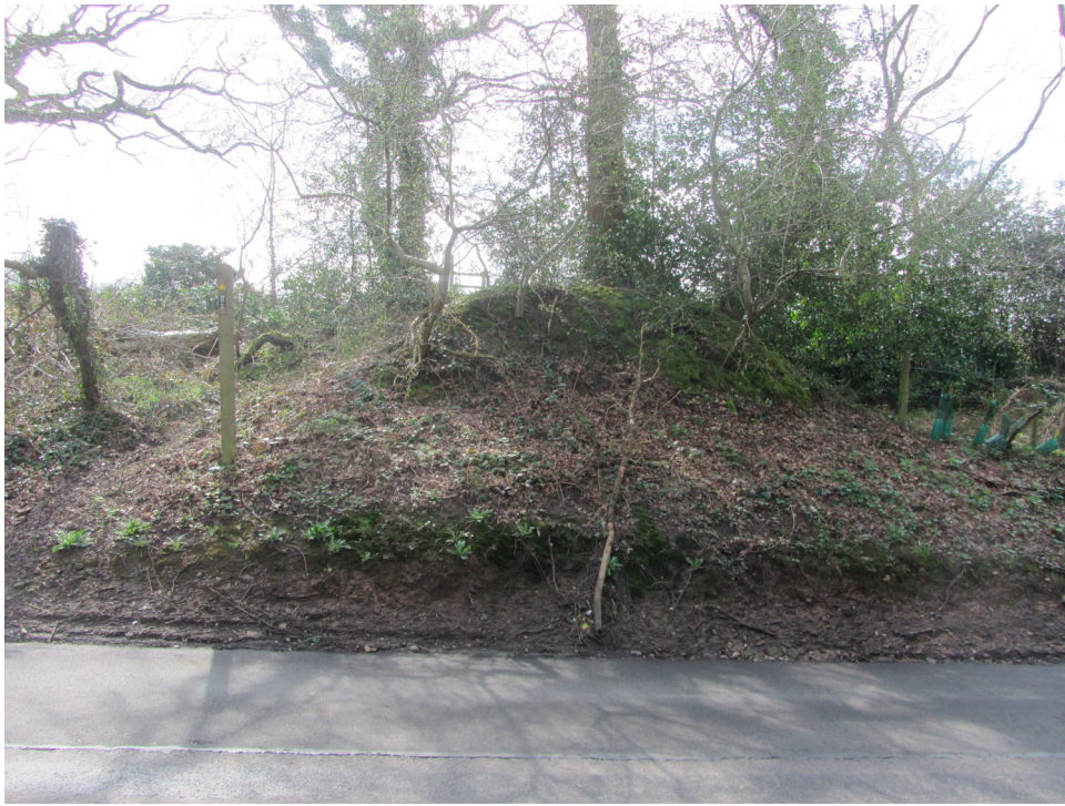
Figure 4. Prior to running alongside the stream, on its route toward the coal yard, the Congleton Railway must once have crossed Mow Lane. The crossing is thought to have been upon a wooden bridge. On the south side of the road this embankment forms a conspicuous feature and must once have formed the approach to the road crossing.
