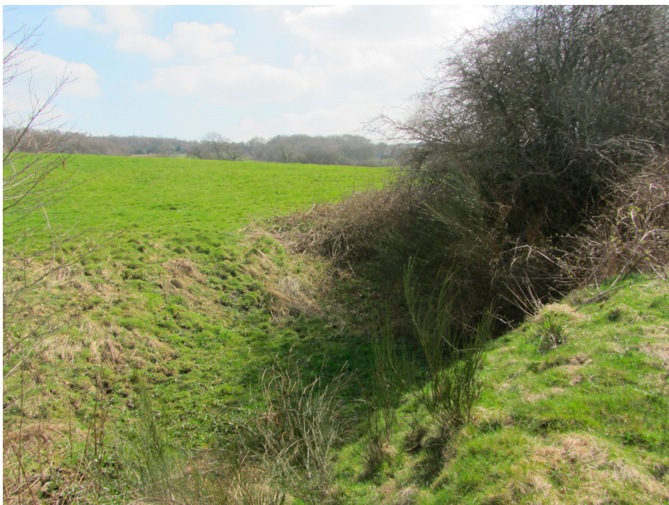
Figure 5. This substantial cutting, seen looking south in April 2018, runs through the fields to the north of Mow Lane and formed the approach of the railway to a crossing over the stream. After this it ran alongside the watercourse on an embankment.
