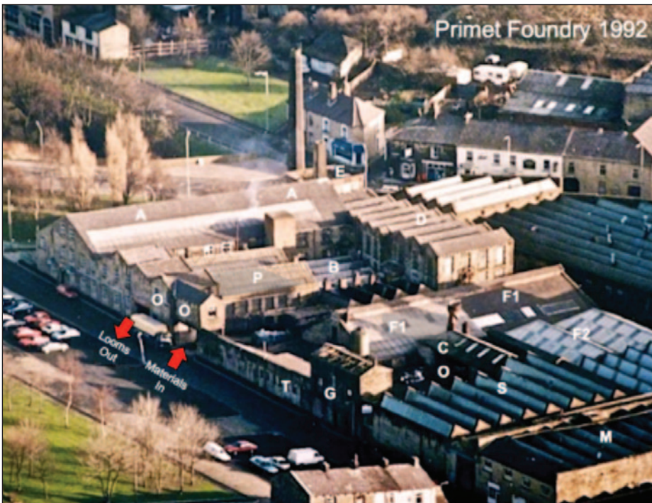
1849 Assembly Shops: 2nd Joinery & pattern shops, 1st Fitters' loom assembly shop, 4th Machine shops, L Gnd Parts & Pattern store 1849 Beam Engine & Boiler. B – Blacksmiths – 7 Forges, plus Furnace. C – 2 Cupolas (Iron Furnaces). D – 2nd Dobby Sley & Electric Motor shops, 1880, 1st Paint shop & bolt store, Gnd Pattern stores fettling & grinding shops, 1857. E – Gnd Engine room for former 200hp tandem compound & generator 1904, Roof tank for Y&T boiler 1895. F1 – Foundry 1857, with sand stores and core oven, F2 – Foundry 1877, F3 – Foundry extended 1895, with Brass Foundry. G – Garage & pattern store, previously 1857 stable, hayloft & horse lorry store. M – 1st Mill – former bridge link to show room from Riverside Mill 1906, Gnd Riverside Mill Warehouse. O – Offices 1877 & 1930, Drawing Office c.1931 Adjacent Silk Shop. P – 1st Packing shop 1947, Gnd Machine shop extended 1895. S – Silk loom shop, former shell shop, R&D / Showroom c.1898. T – Timber saw pit 1857 original fire proof store, then from 1952 WCs
