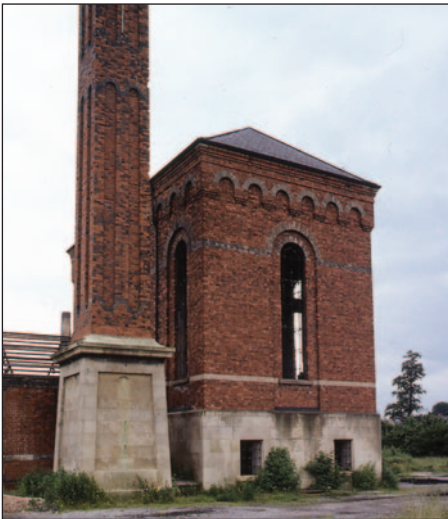
Bracebridge Pumping Station, Worksop, 1980 photo Amber Patrick
