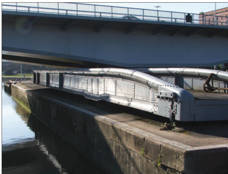
West end view of Brunel's other Bridge with Plimsoll Bridge above
