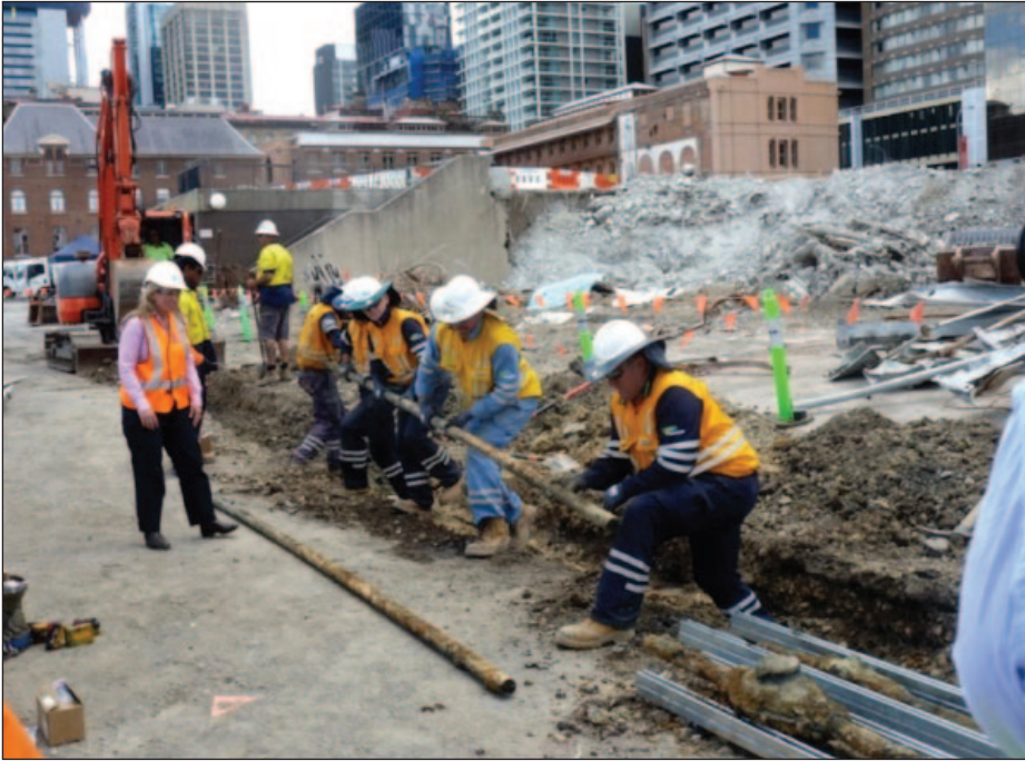
The 2018 dig in William Street. Careful removal of full 20 feet lengths of Edison Street Tubes from the excavation photo: Brian Becconsall, February 2018.
