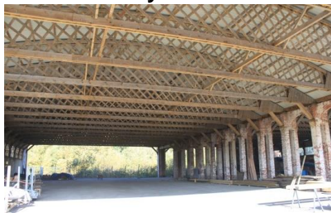
Belfast Trusses at Hooton Park
