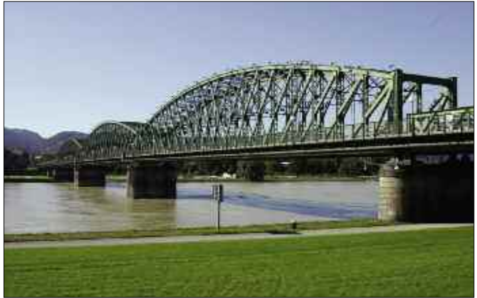
Linz railway bridge
