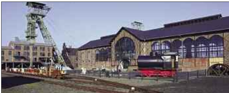
Erected in Dusseldorf for the 1902 Industrial Exhibition, the Zollern machine hall was dismantled and moved 100 km to Dortmund where it was re-erected with the famous Jugendstil entrance. Photo: LWL – Industriemuseum
