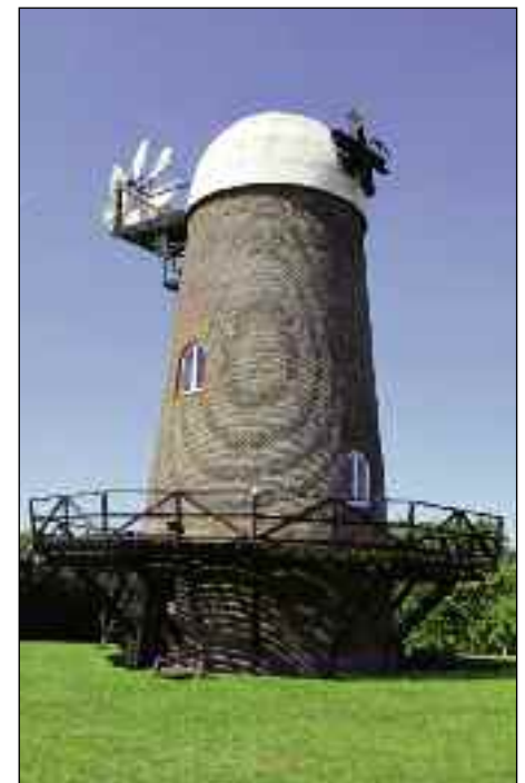
Wilton Windmill after the sails were removed for repairs in August 201
