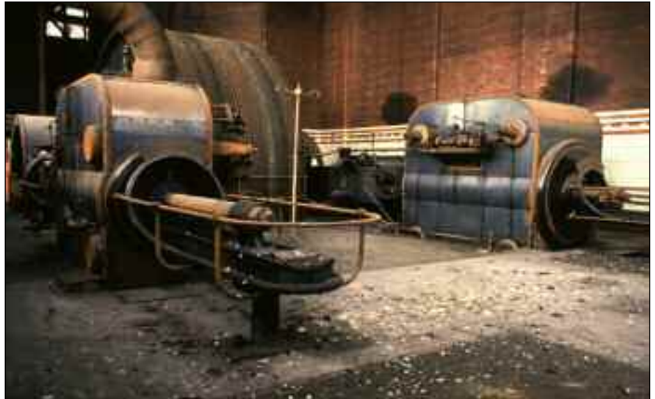
Leigh Mill engine after building weatherproofed
