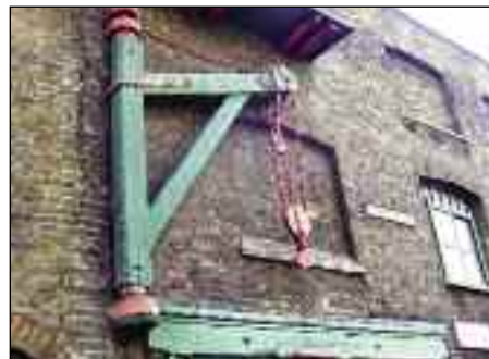
Rare timber wall crane
