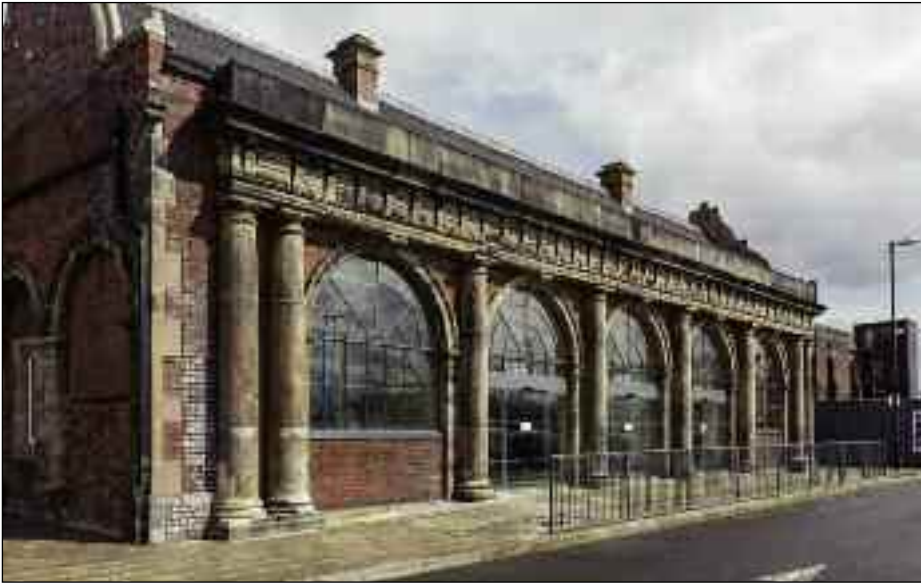
Stoke on Trent downside entrance
