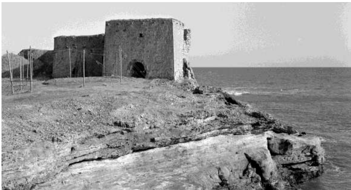
Fig. Boddin Limekilns in Angus after a major collapse (compare 1993 photo in gazetteer) but before some more recent erosion, with drying poles for Usan Fisheries. This illustrates rough terrain and a need for caution (Ted Salthouse, SIHS)
