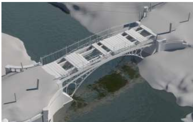
Below, Linlathen East Bridge, before repairs, derived from digital scanning by CDDV
