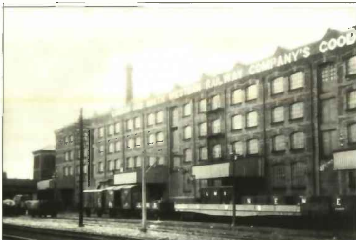
SK21: London & North Western Railway Company Goods Warehouse, Heaton Norris.
