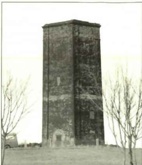
W116: Wall Hey Pit Ventilation Shaft Chimney.
