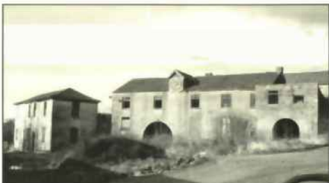
BO18: Wallsuches Bleach Works.
