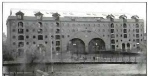
M27: Middle Warehouse with shipping holes and elliptical arch, Castlefield. Photo Steve Stockley
