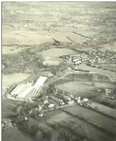
BU09: Stormal Hill Bleach Works and Tottington Viaduct. Photo Barri Jones © GMAU
