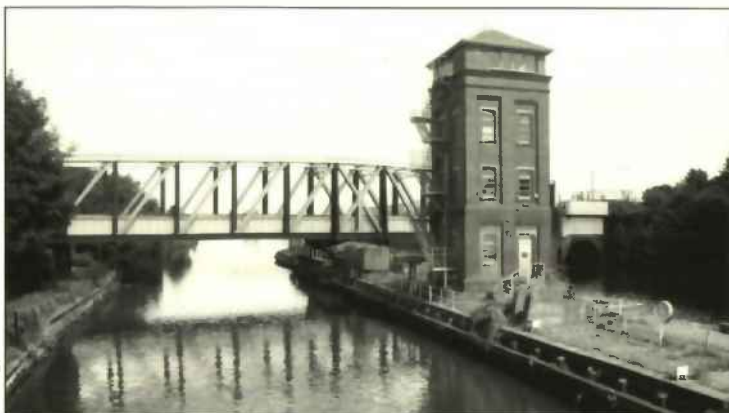
SA31: Barton Tower and Swing Aqueduct
