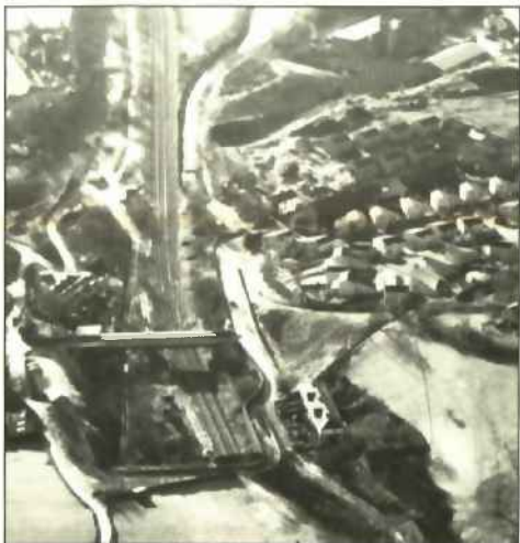
OL38: Diggle Tunnels for the Huddersfield Canal and Railways. Photo Barri Jones © GMAU
