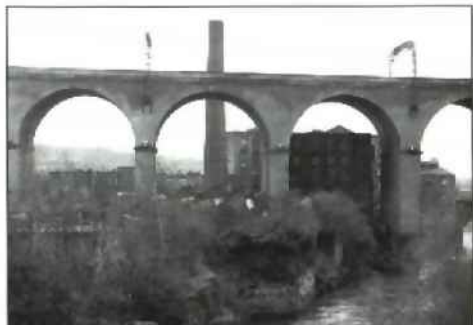
Stockport Railway Viaduct.
