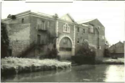
TR19: Canal Warehouse, Broadheath
