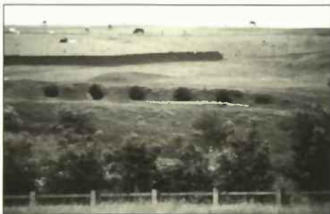
RO20: Tunshill Coke Ovens
