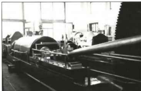
RO09: Ellenroad Engine House
