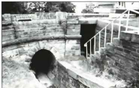
SK17: Rossett Bridge Horse Tunnel, Peak Forest Canal. Photo: Arthur Clarke
