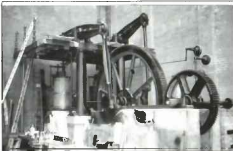
BO9: Beam engines - Northern Mill Engine Society Museum. Photo David Lewis
