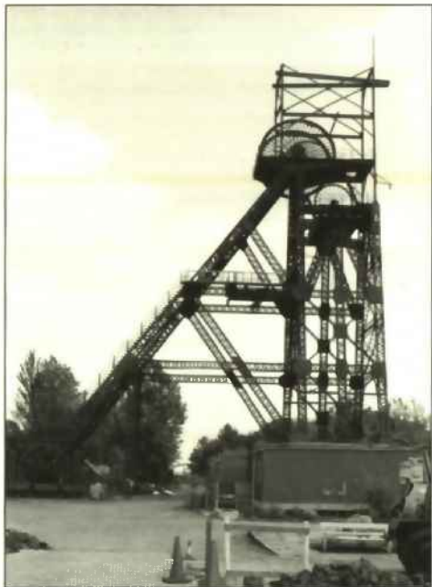
W114: Astley Green Colliery Pit Head
