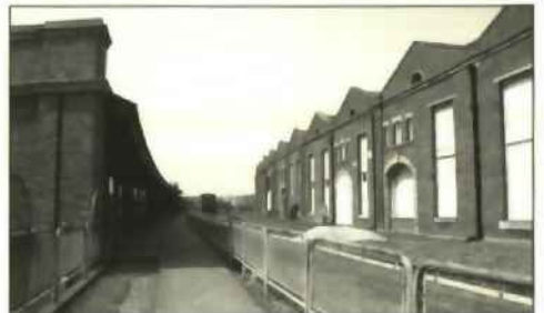
M40 Liverpool Road Station and Warehouse
