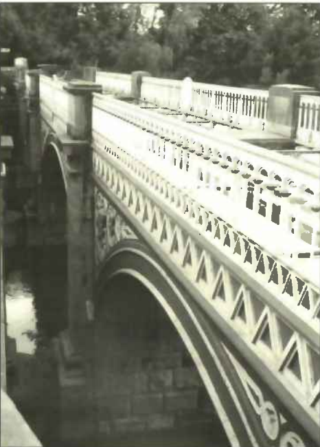
BU25: Thirlmere Aqueduct
