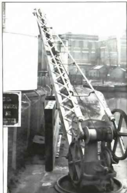
SA31: Stop Plank Crane Bridgewater Canal at Barton Aqueduct. MRIAS archive
