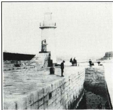
W11.5: West Pier and Lighthouse, Whitehaven
