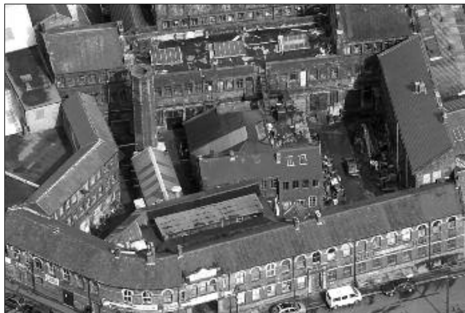
Portland Works, Randall Street, Sheffield
