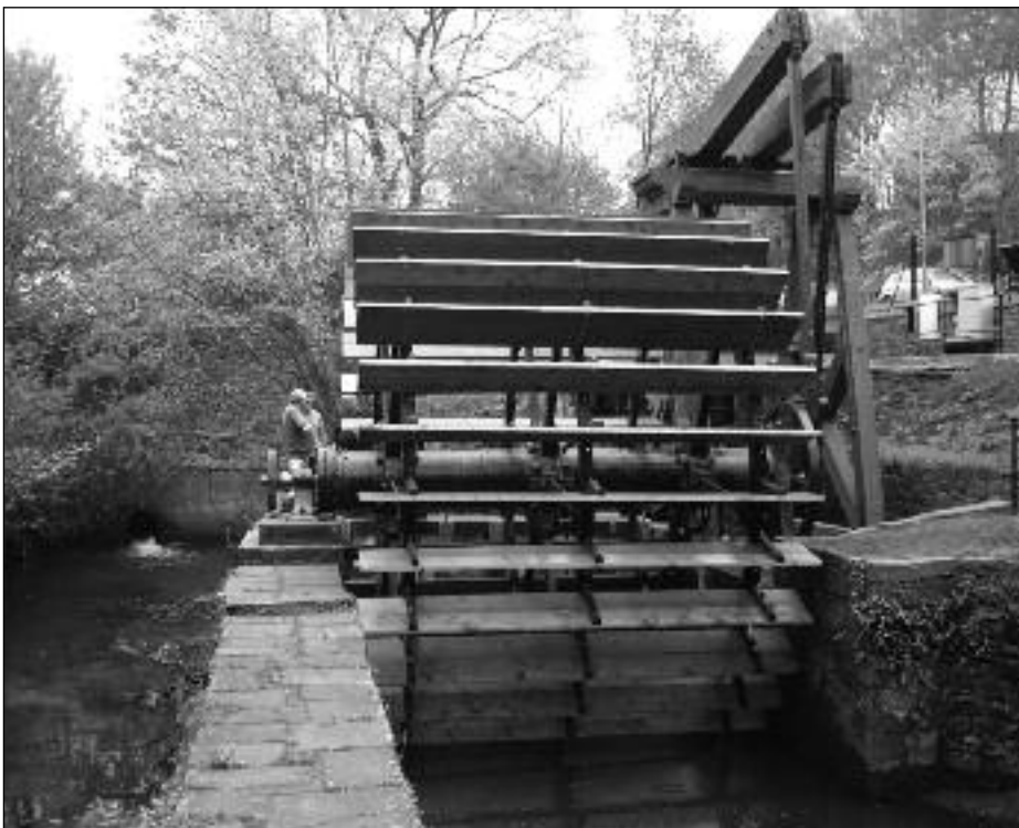
Melingriffith Wheel looking upstream showing the tailrace exiting the tinplate works site. The original wooden dam was on the left to raise the level of water to drive the wheel Photo: Stephen Rowson
