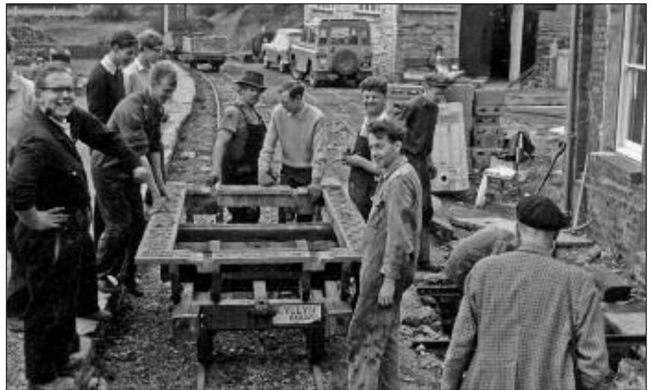
Tallyllyn Railway Weighbridge removal 1964
