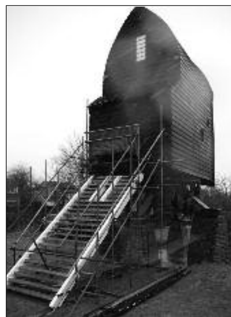
Chinnor Windmill new ladder installed
