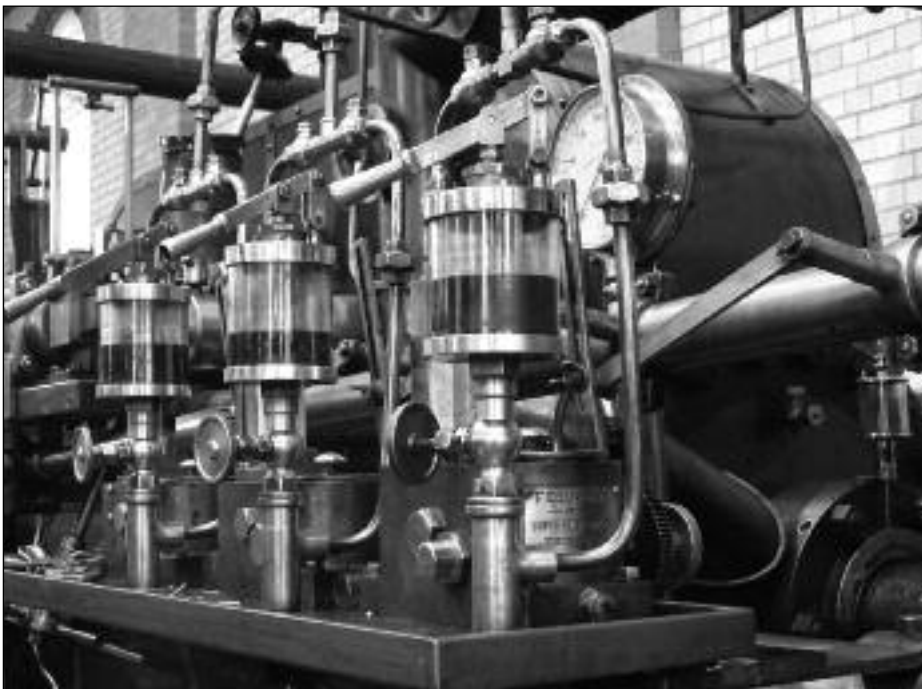
Mill Meece Pumping Station
