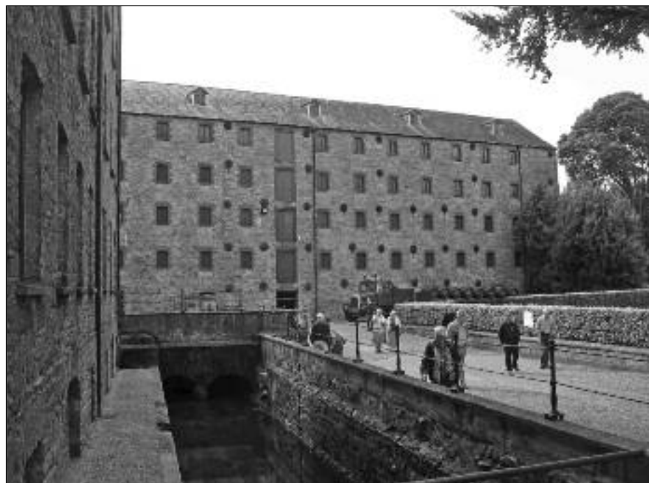
Jamesons Midleton Distillery Warehouse
