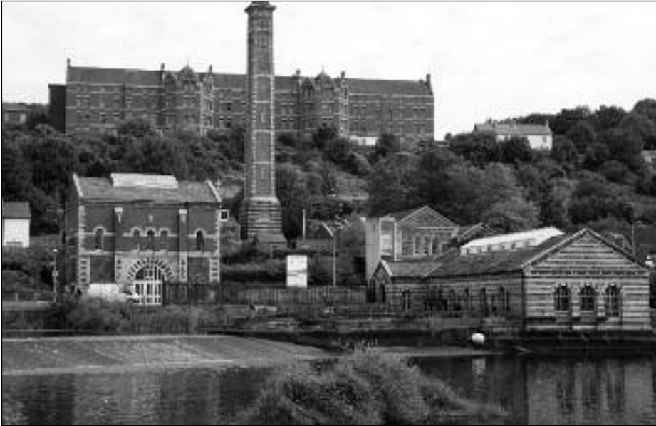
Cork City Water Works with County Asylum behind
