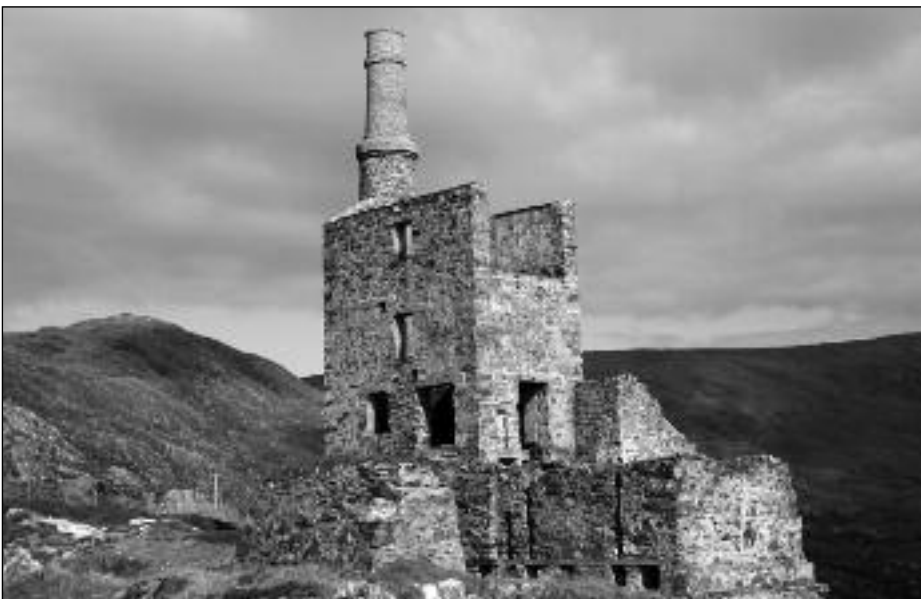
Restored Man-Engine House at Allihies Copper Mine
