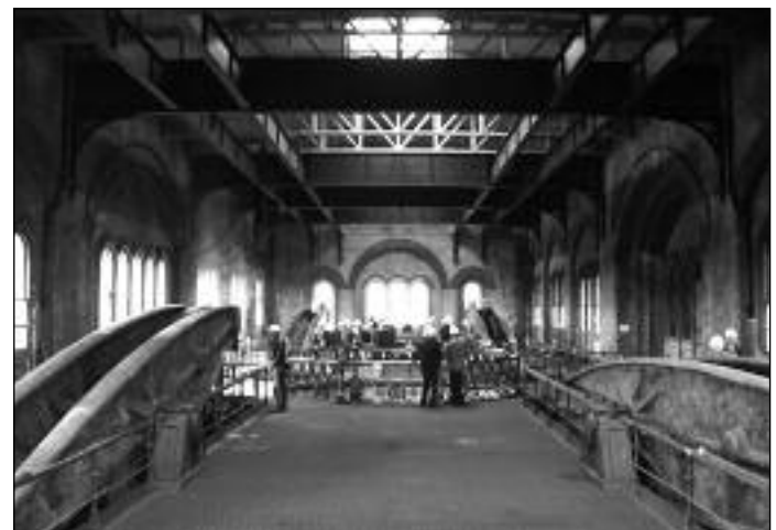
Crossness Pumping Station, Bexley, London
