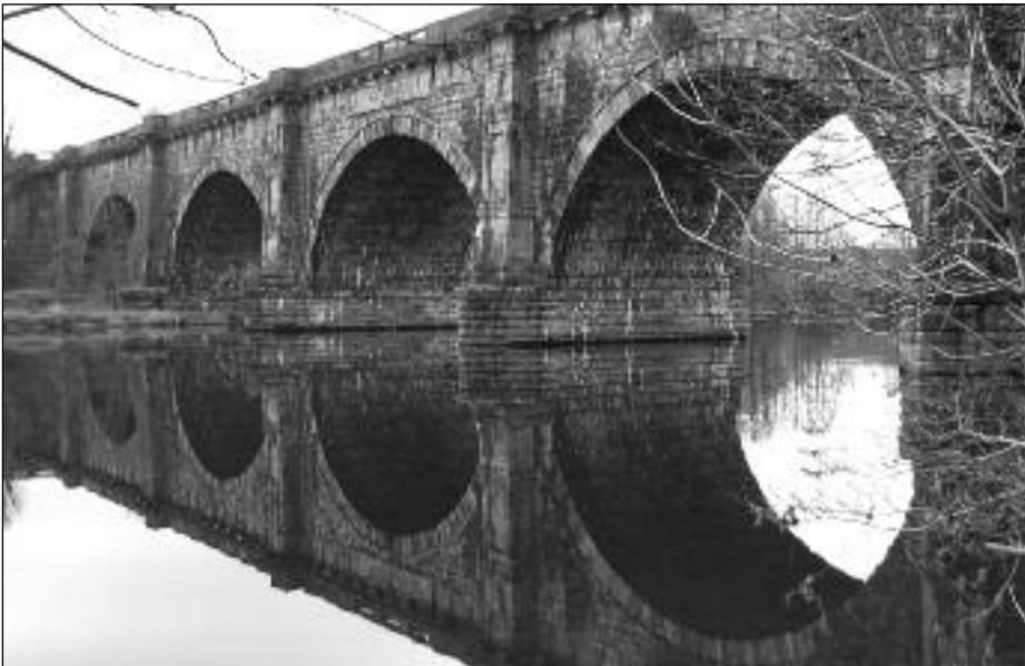
Lune Aqueduct on the Lancaster Canal
