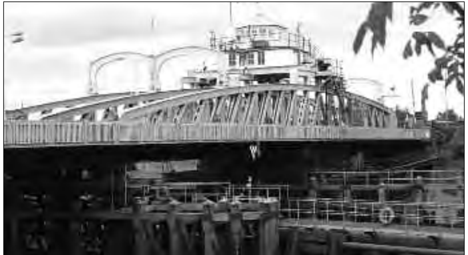
The swing bridge at Sutton Bridge across the navigable and tidal River Nene
