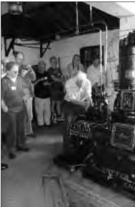
Starting the Petters diesel at Gayton Engine Pumping Station Photo: Steve Dewhirst
