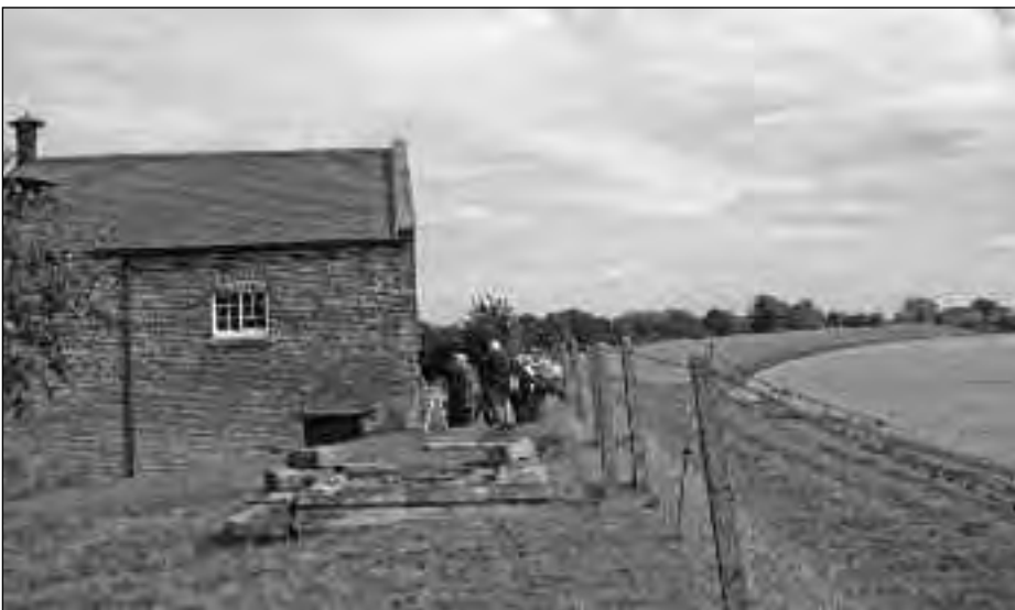
Dogdyke pumping station beside the River Witham
