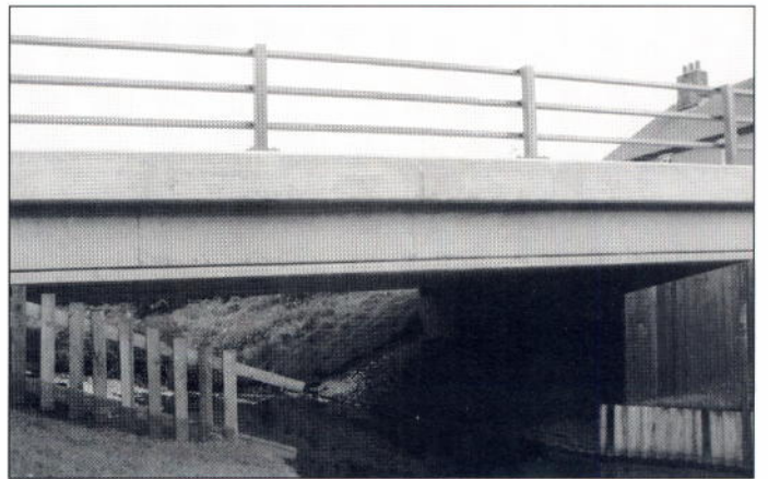
Banningham Bridge, as rebuilt in 1994-5. West elevation
