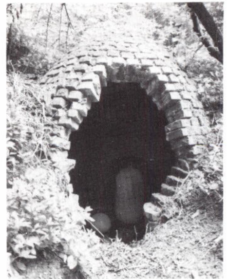
The ram and beehive ram house of c1845 at Ossington Hall, Newark Photo: The National Trust
