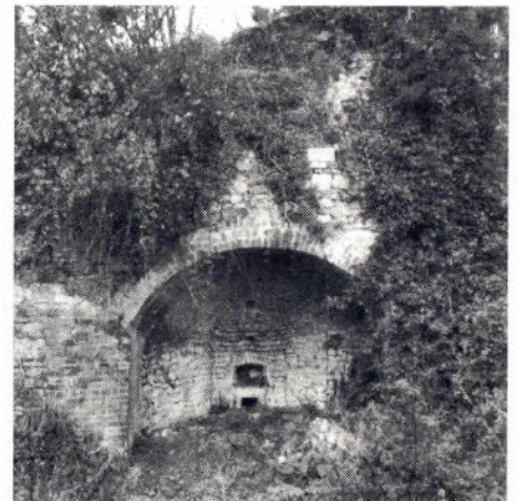
above left: Limekiln with round draw arch in stone (type A) at Longburton, North Dorset above right: Limekiln with pointed draw arch (type C) at Loders, West Dorset below: Limekiln with round brick draw arch (type B) at Woolland, North Dorset
