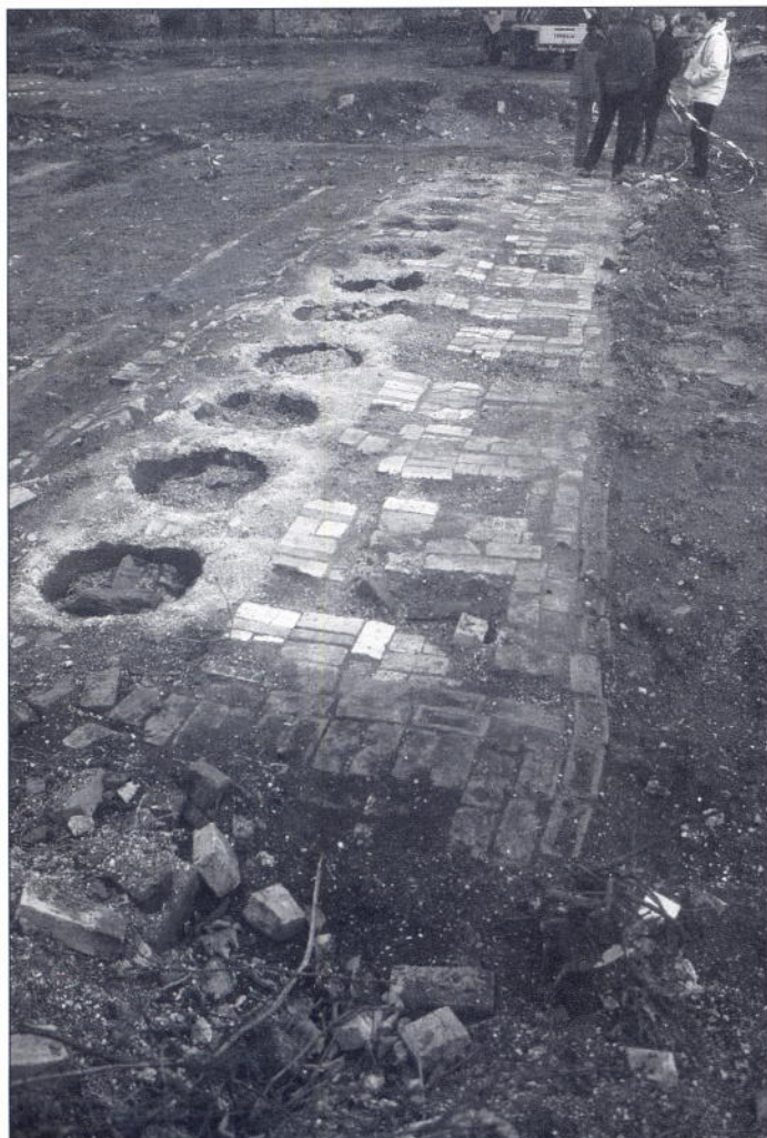
Crucible holes at the Wadsley Bridge steelworks site
