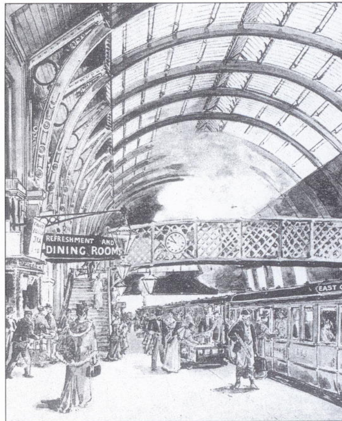
Platform 8 at King's Cross in the 1890s, looking north. The Flying Scotsman will depart shortly
