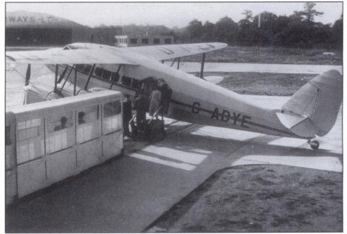
Gatwick passengers boarding a DH86 aeroplane in 1936 by means of a telescopic corridor
