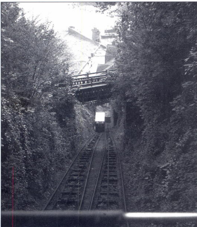
Powering the Lynton & Lynmouth cliff railway in north Devon is one unusual application of water described in last year's Dorset water conference
