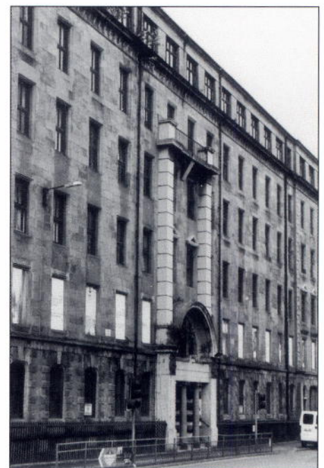
R. F. & J. Alexander's cotton thread mill of 1849, Glasgow, converted to the Great Eastern Hotel by additional top storey and entrance alterations, 1907-9
