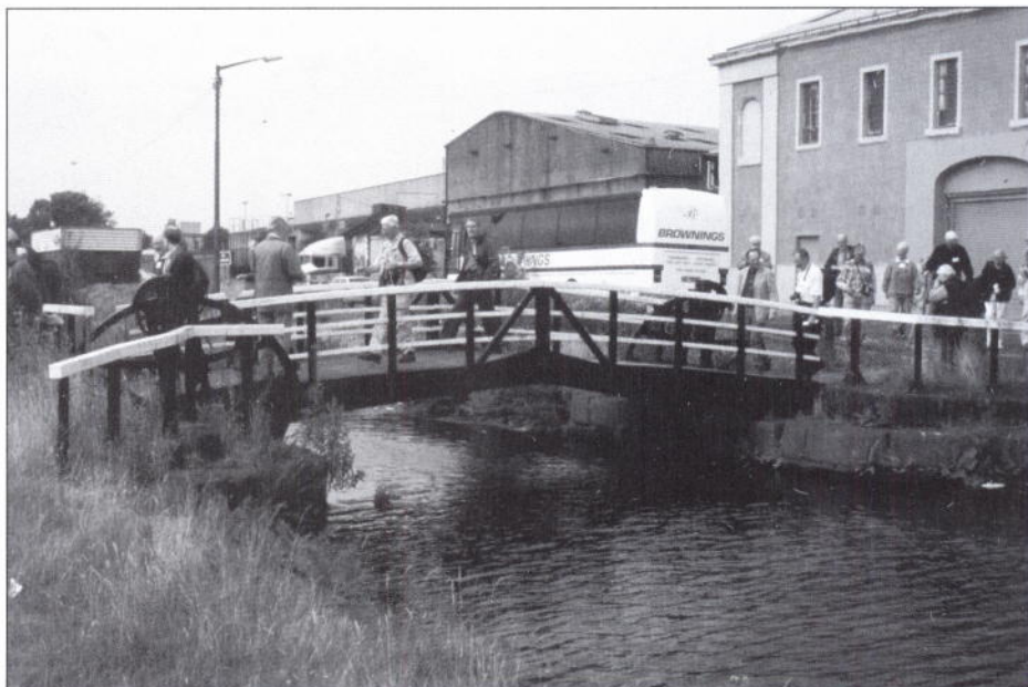
Delegates crossing a replacement twin-leaf lift bridge over the canal at Spier's Wharf North, Port Dundas, Glasgow
