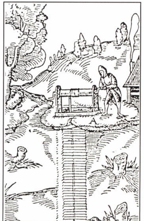
Winding at a German mineshaft, from Agricola, De Re Metalica , 1556
