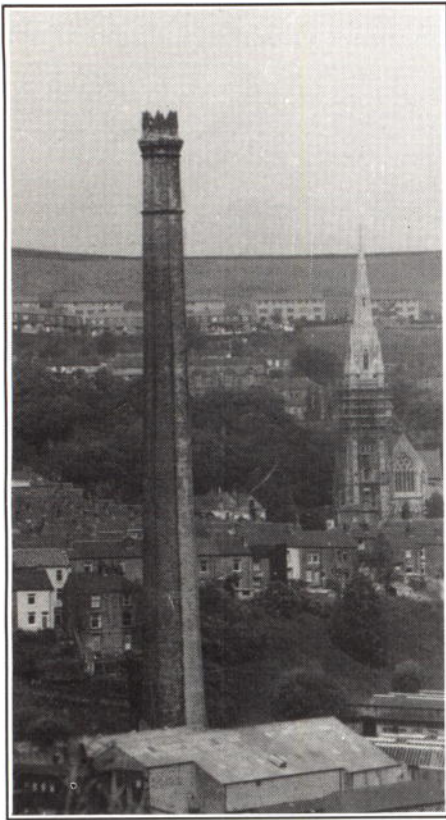
Dean Clough Chimney, Halifax, 1857
