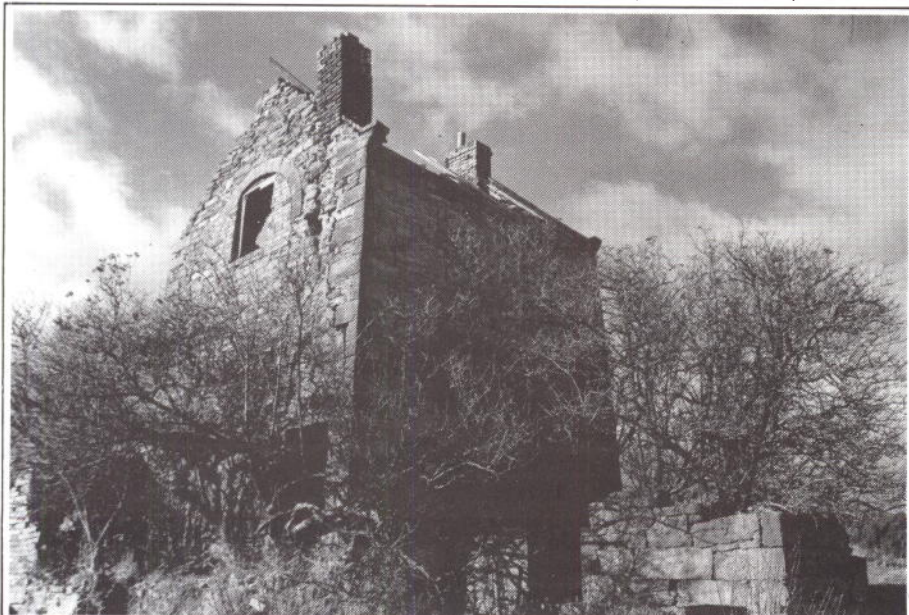
Beam-engine house at Penrhos, Clwyd (SJ 286532) built by John Wilkinson c1794 and later converted to a dwelling. The building was recognised during research for a new gazetteer (see appeals for information). The bob wall and arch and the chimney are shown.
