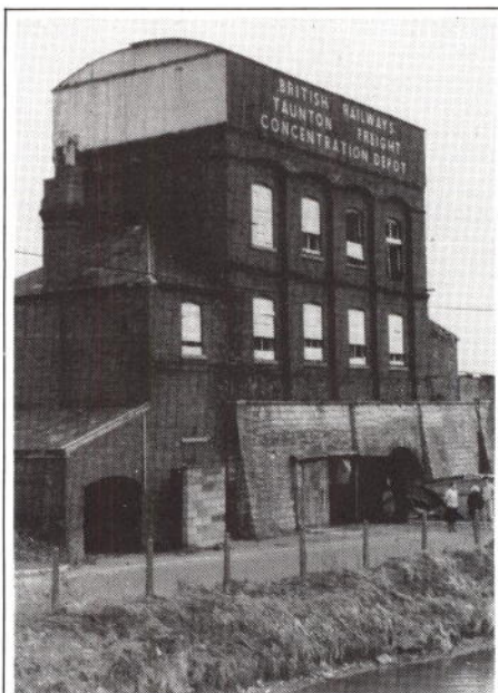
Canal frontage showing the limekilns from the 1840s with the pumping house and water tank superimposed.
