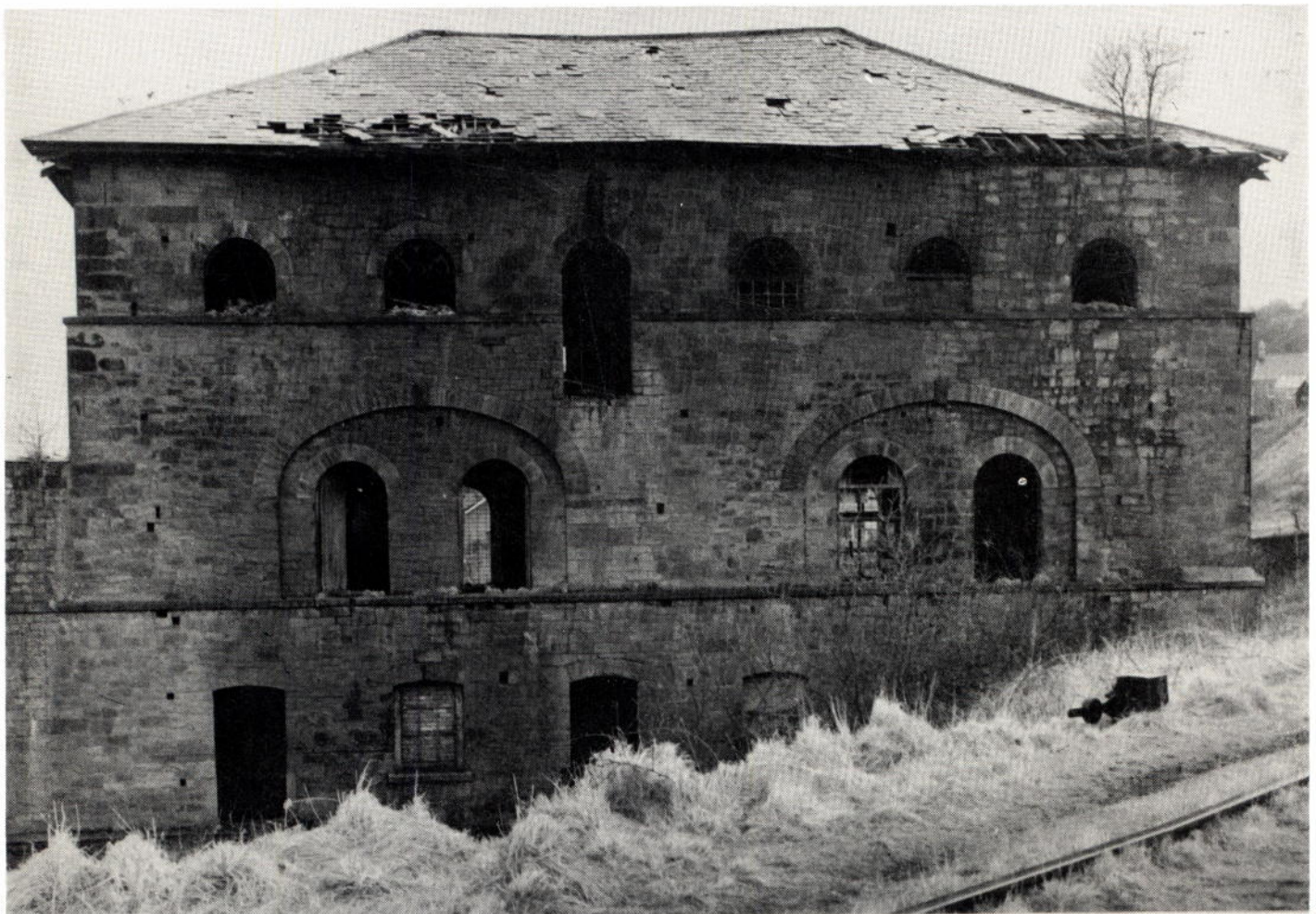
The great engine house at Maesteg
