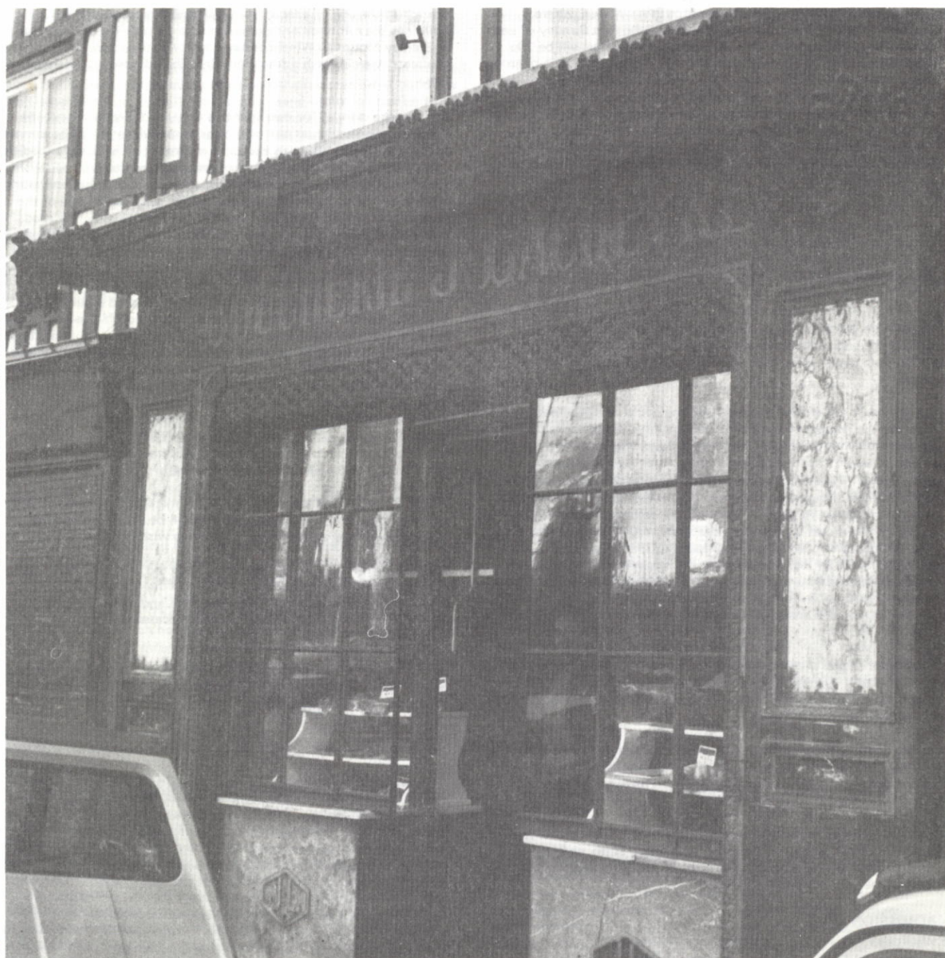
Typical 19th century French cast iron shop front, inset with marble panels. Photographed at Harfleur, Normandy, January 1977.
