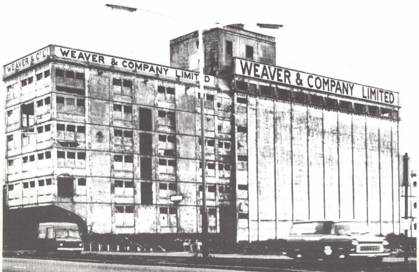
Weaver's Warehouse at Swansea
