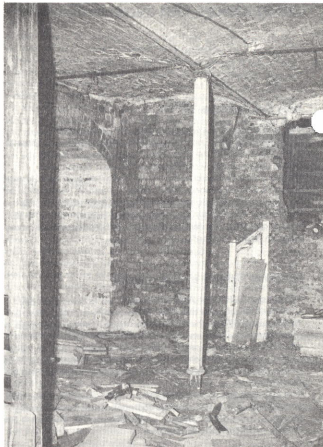
Cellar of same house.
