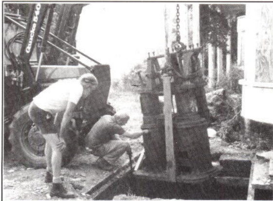
The Taplow engine being rescued from its cellar
