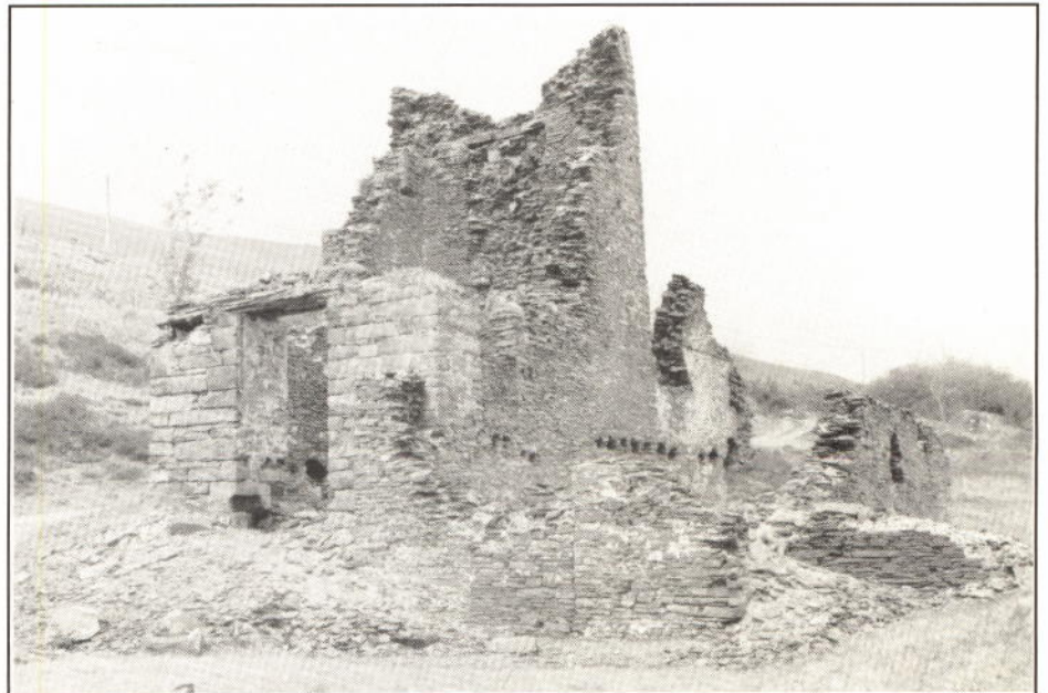
The Crusher house at Frongoch lead mine, in 1984; see Welsh Mills Group , page 6
