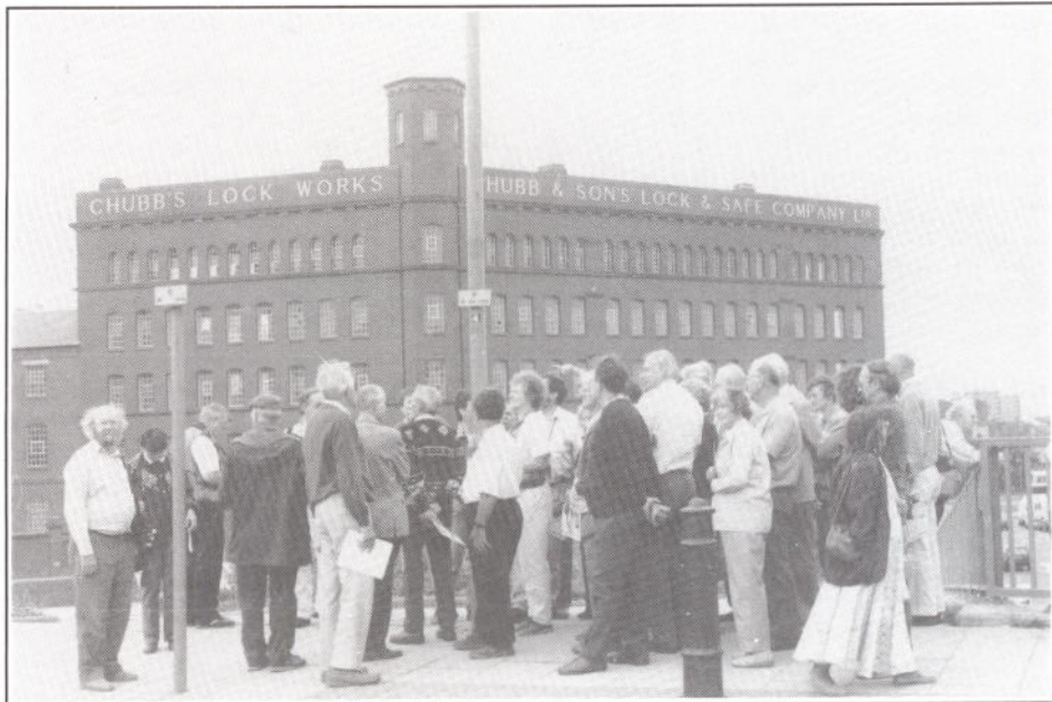
The Dudley Conference: exploring the Iron District (see page 2-3). The former Chubb works in Wolverhampton, built in 1899, during conversion to a media and arts centre Photo: Marilyn Palmer and Peter Neaverson
