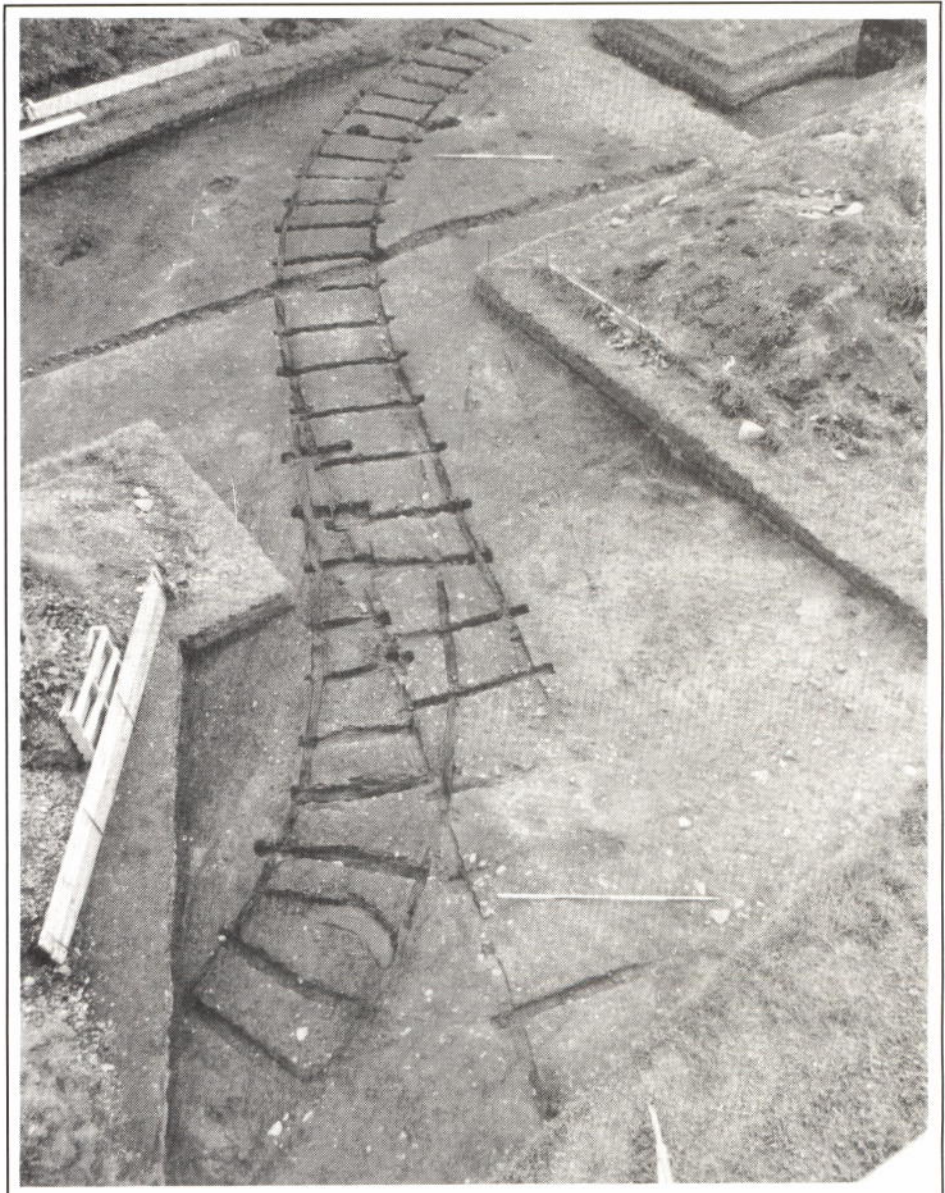
Wooden waggonway at Bersham: the track and points after excavation and removal of the carbonised timbers Photo: Stephen Greuter
