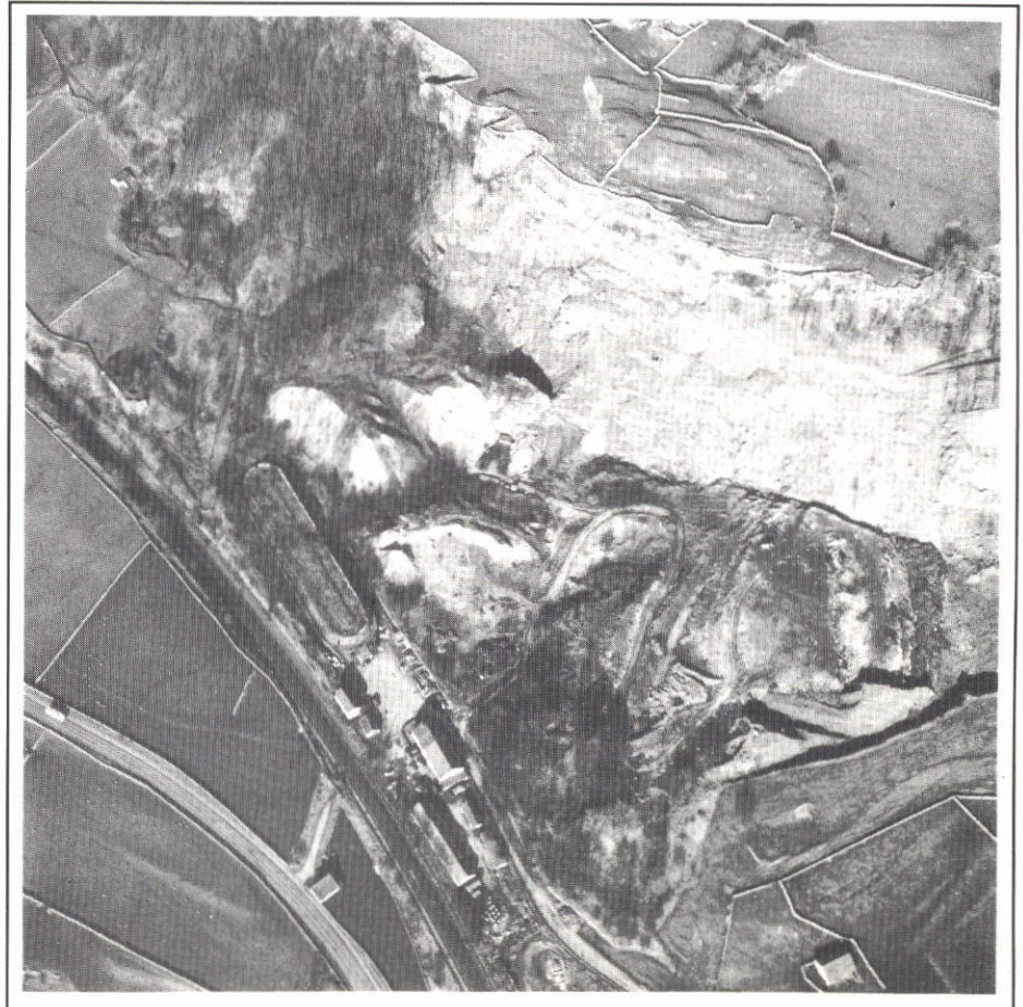
Aerial view of the Langcliffe limeworks
