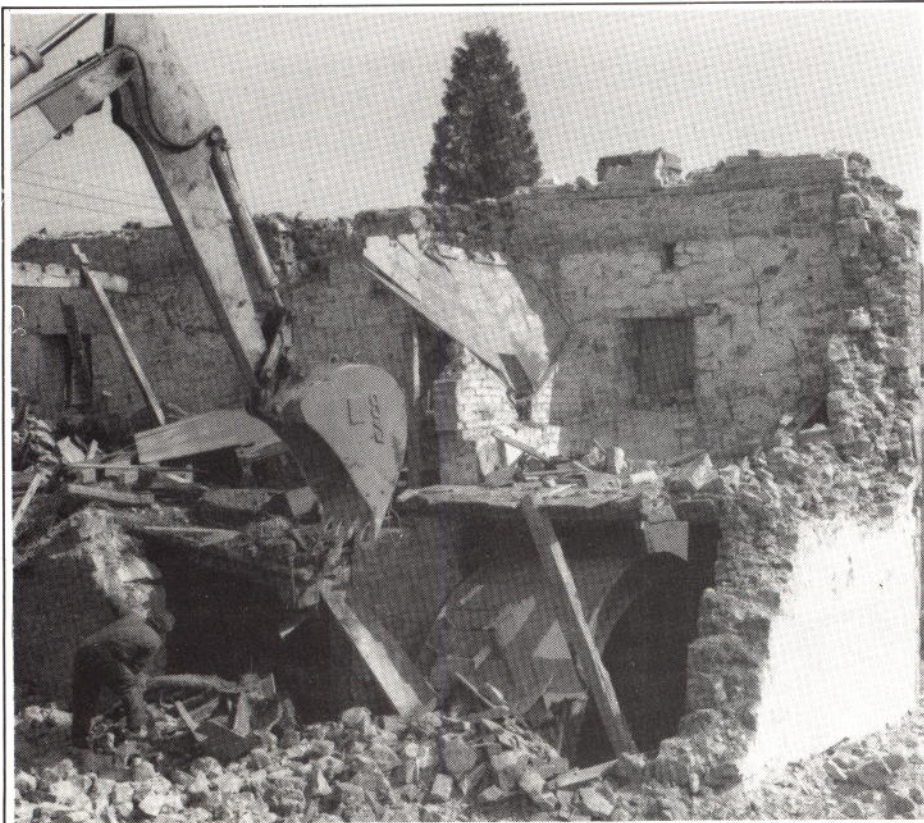
Destruction in Wales: White Mill during demolition, showing the pitch-back wheel, one of the stones and the remains of grain hoppers Photo: © National Monuments Record for Wales
