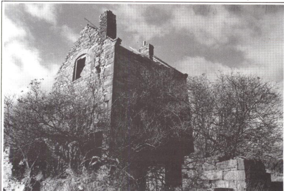
Beam-engine house at Penrhos, Clwyd (SJ 286532) built by John Wilkinson c1794 and later converted to a dwelling. The building was recognised during research for a new gazetteer (see appeals for information). The bob wall and arch and the chimney are shown.
