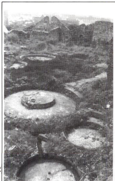
2. Concrete centre-head buddle, West Basset, Cornwall, 1875
