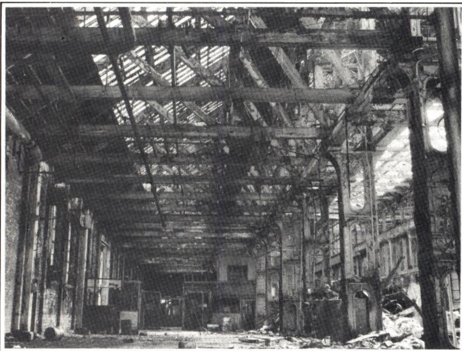
The interior of the 1872 Engine Shop at Alexander Stephen's Linthouse Yard.
