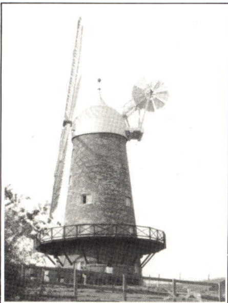
Sneinton Windmill after restoration.
