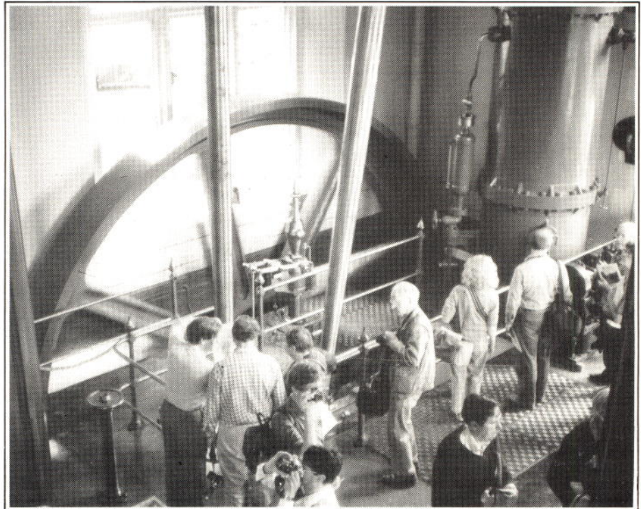
Preserved 1902 Glenfield and Kennedy Beam Engine at Bristol Waterworks Company's Blagdon Pumping Station.
