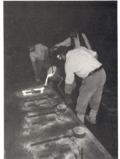
21st June 1985, the first 'cast' of the new Blists Hill iron-foundry.
