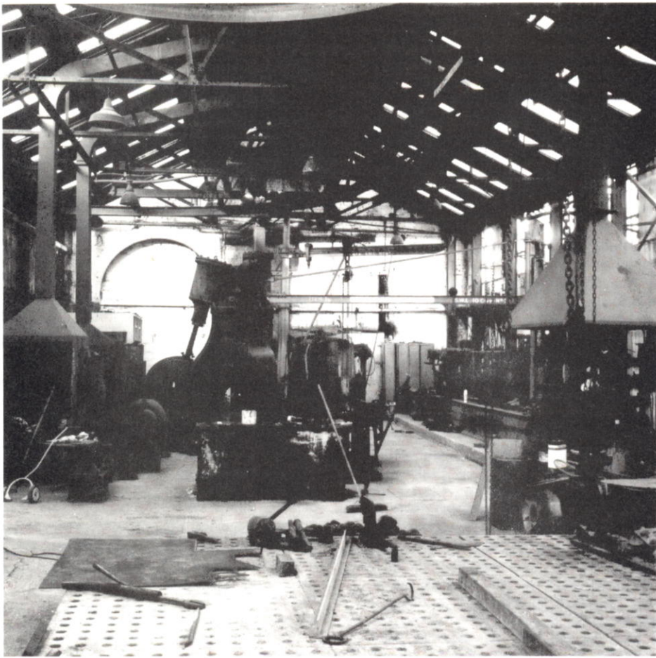
The Blacksmiths' Shop at the West India Dock Works of River Thames Shiprepairs Ltd in 1980. This view, looking north, shows a pneumatic hammer by B & S Massey of Manchester and forge hearths. In the foreground is a rib bending floor. The furnaces which heated the ribs before they were worked upon are behind the camera. Technology similar to that which this photograph illustrates was practiced in the 1860s when the shipbuilding industry on the Thames declined. The forge shown in the above view was cleared of its machinery and fittings soon after the photograph was taken. It would only be practical to establish a fully representative ship-repair yard museum including large machines by preserving a closed yard in situ.
