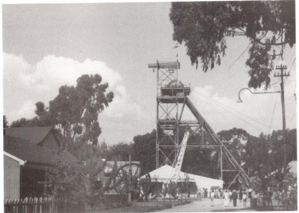
Headframe of No 14 shaft, Crown Mines Museum.
