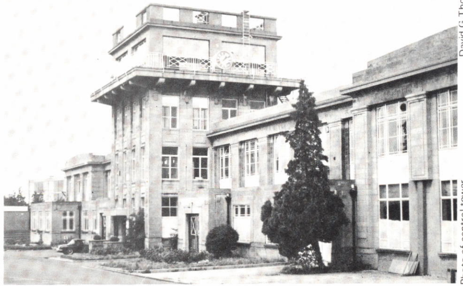
Photo of control tower David G Thomas
