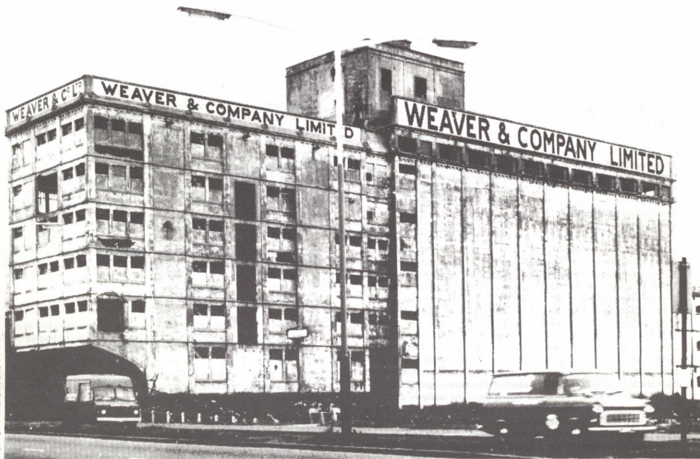
Weaver's Warehouse at Swansea
