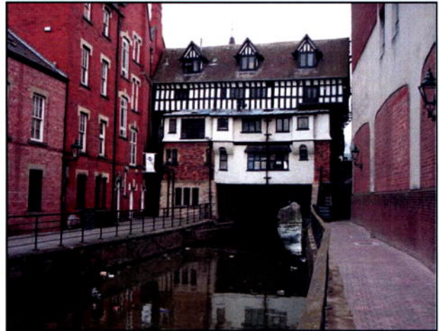
Figure 2: High Bridge, Lincoln
