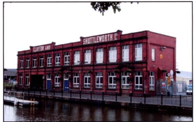
Figure 5: Edwardian office block of Clayton & Shuttleworth's Stamp End Works, Waterside South
