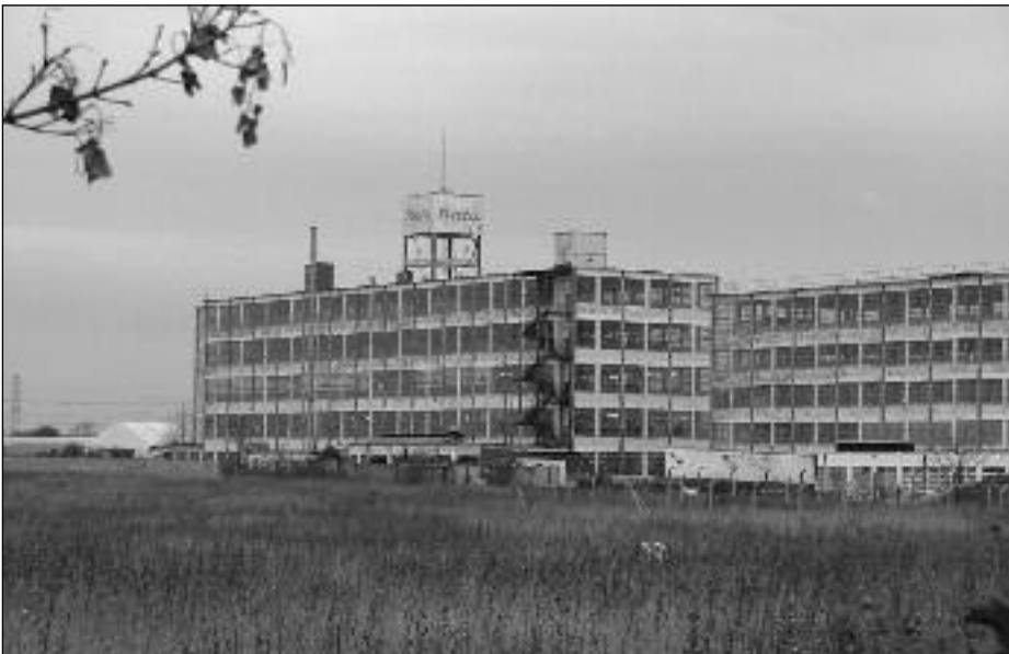
Bata Factory derelict buildings
