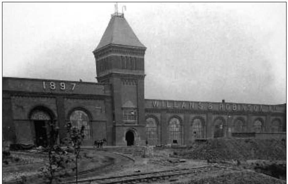
Willans and Robinson Works under construction in Rugby – much of this survives
