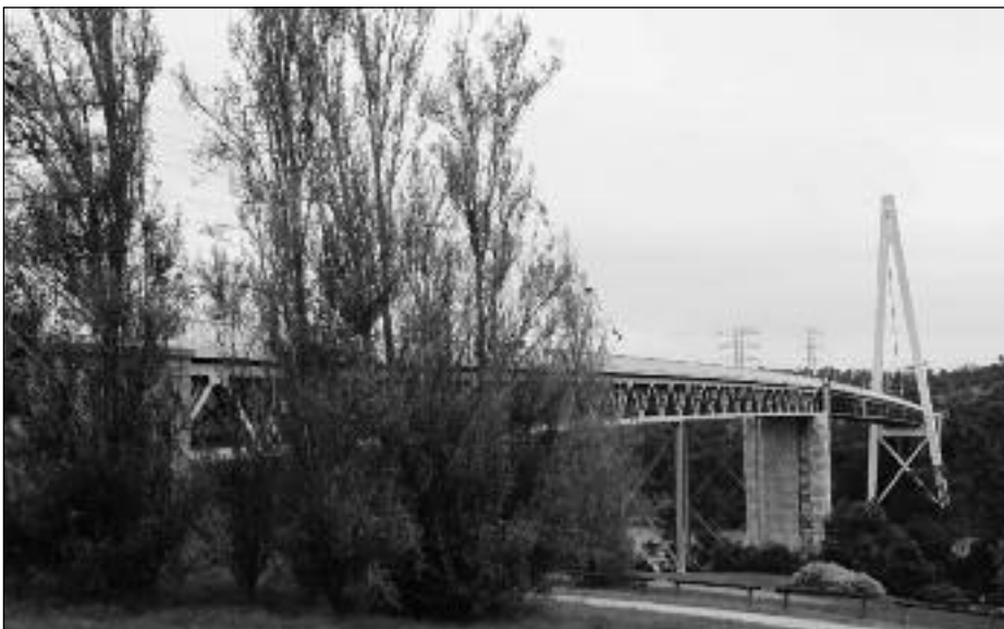
260m span Batman Bridge crossing the Tamar River, Tasmania. The first cable stayed bridge in Australia, built in 1966
