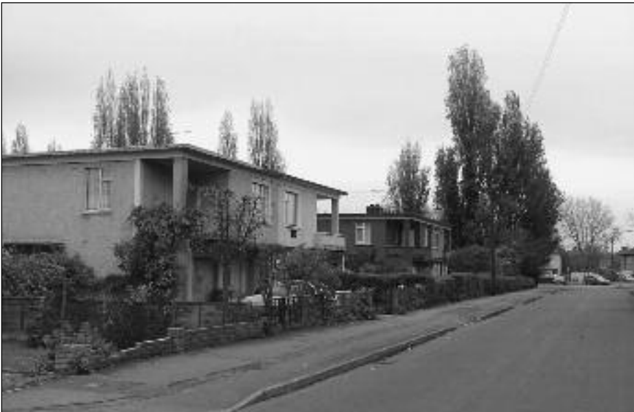
Bata Manager's House
