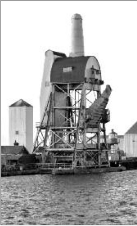
Goole Tom Pudding Hoist
