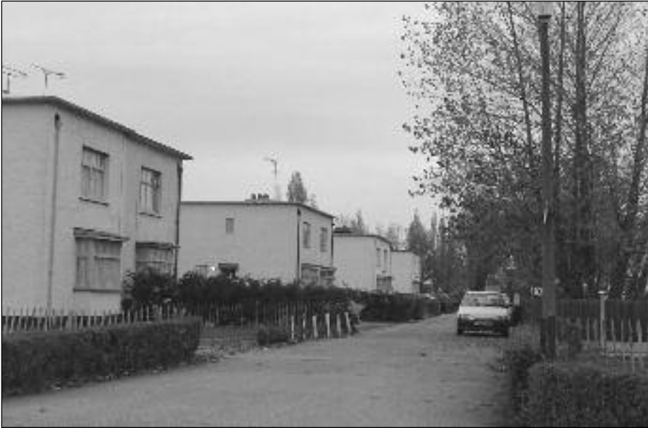
1933 Modernist houses in Bata Avenue
