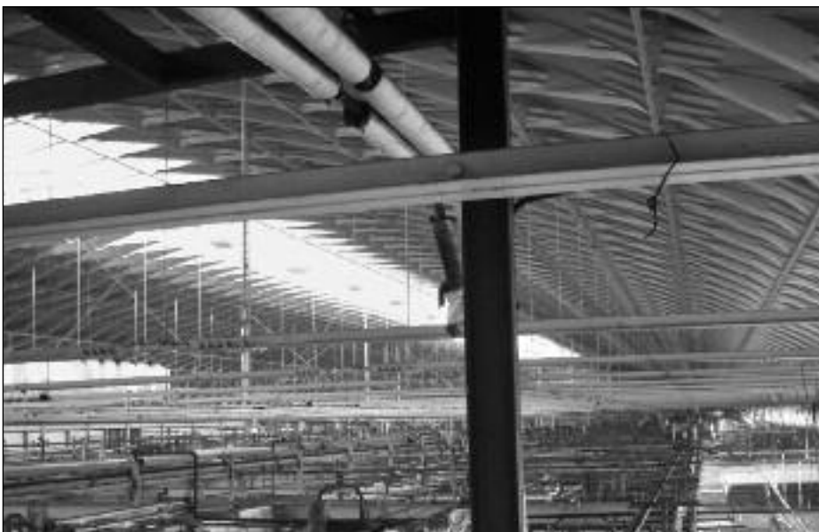
Longbridge Flight Shed roof
