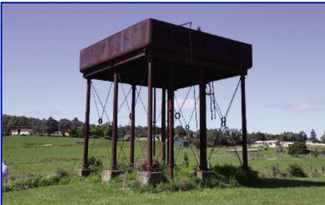
Water Tank at St Mary's, Tasmania, cast in Manchester 1884 by Ashbury & Co
