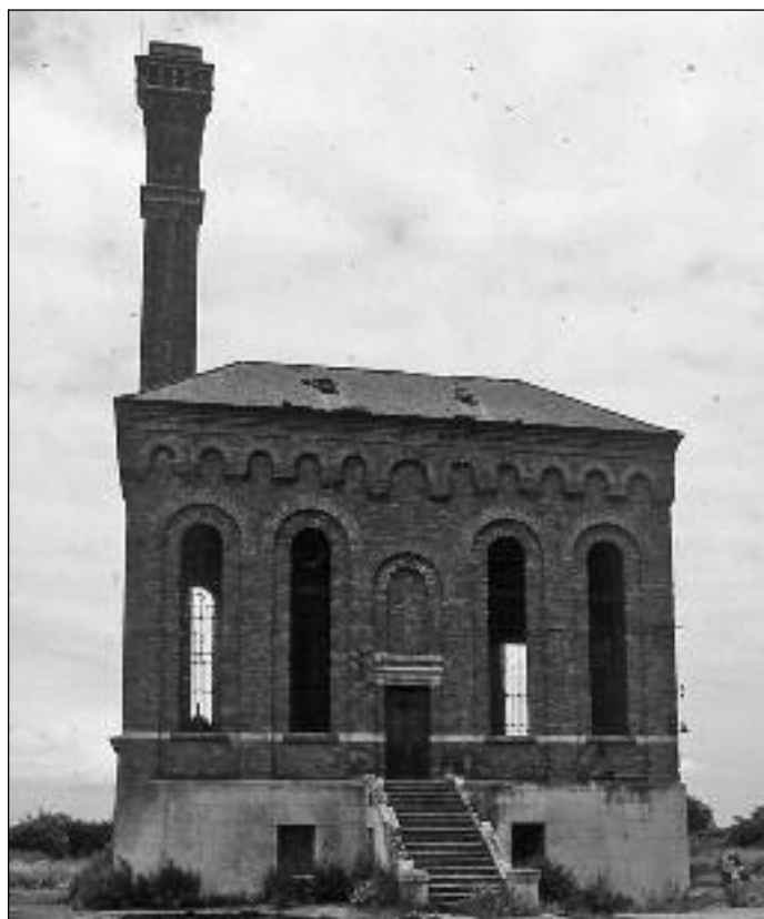
Bracebridge Pumping Station, Worksop 1980
