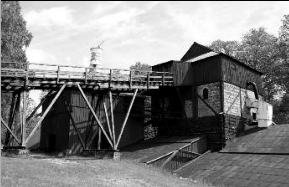
Engelsberg earth and timber blast furnace as reconstructed in 1878. It was last blown in 1919
