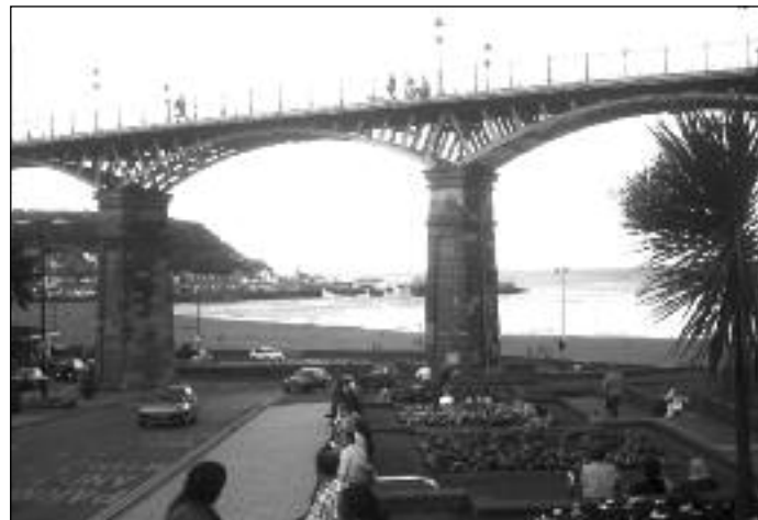
Scarborough Spa Footbridge 1826, widened 1880
