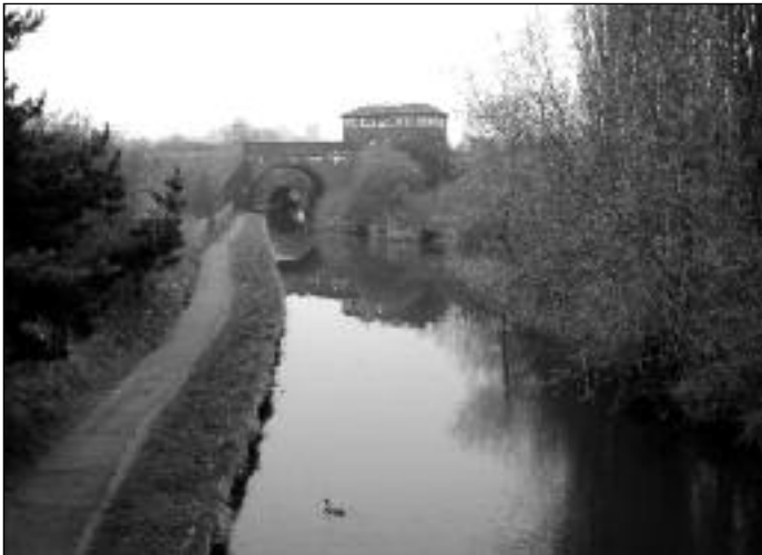
The Droitwich Barge Canal looking towards Netherwich Tunnel, which is now lit for pedestrians. The signalbox indicates a surviving enclave of semaphore signalling Photo: John Powell
