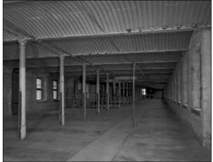
Clocktower Warehouse, Dundee converted to flats: first floor view prior to conversion Photo: © RCAHMS SC1047298
