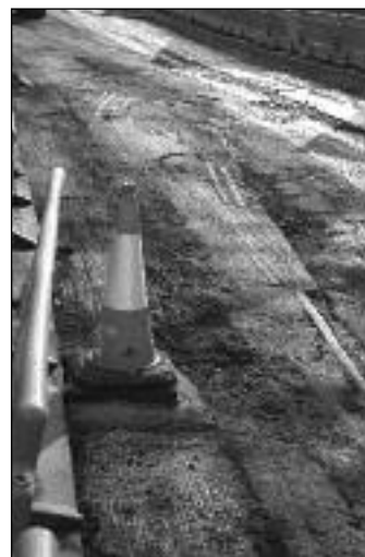
Exposed tramway track in Wantage Photo: Henry Gunston
