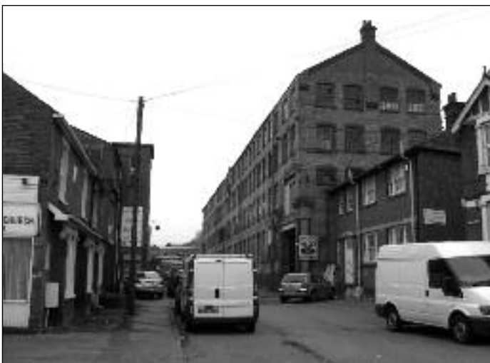
W. Birch Works, Desborough, High Wycombe
