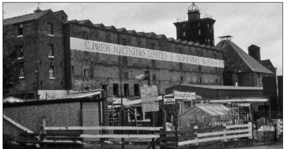
Ditherington Mill as now seen from the road
