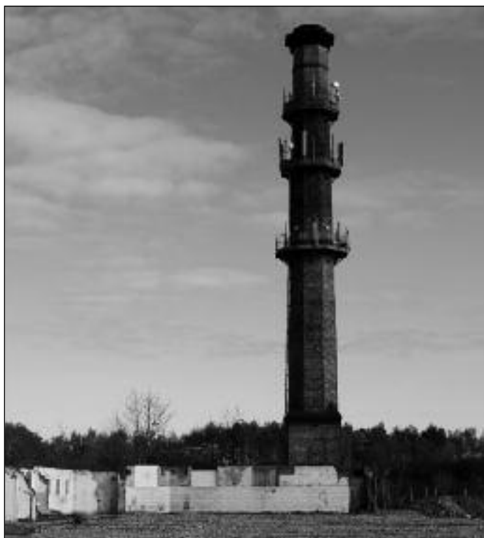
Long Eaton Mill Chimney spared from demolition – reused as aerial
