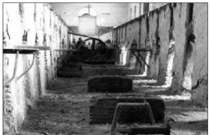
Stripped out line shafting with the main drive pulley
